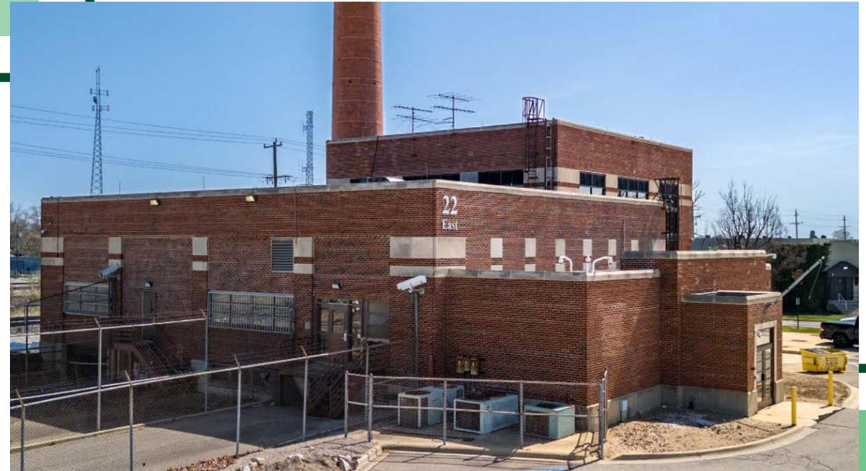
The Central Heating Plant, built in 1947, houses the main north campus steam boilers. The Central Laundry also occupied part of this facility until 1982 when laundry services were contracted to outside vendors. In 1982, a steam efficiency improvement program was implemented to reduce the main loop pressure from 125 psi to 80 psi to conserve energy. In 1986, the laundry portion of the building became the Sheriff's Men's Satellite Facility until early 2010.
