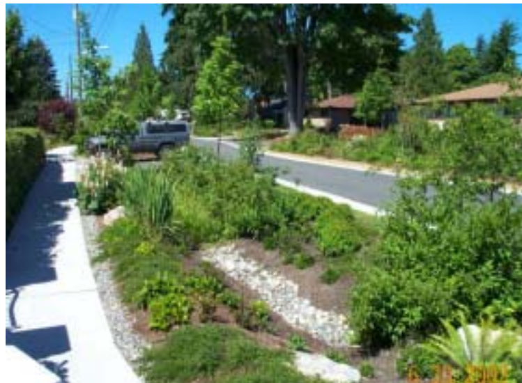
Street-side swales can dramatically reduce stormwater runoff from roads (Photo: Seattle Public Utilities)
