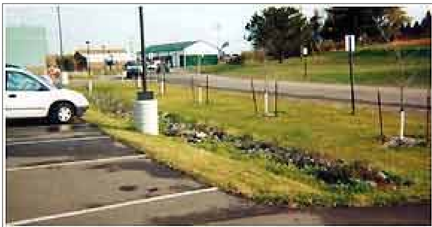
A condensed vegetated filter strip at the City Hall in Proctor, Minnesota (Photo: City of Proctor)
