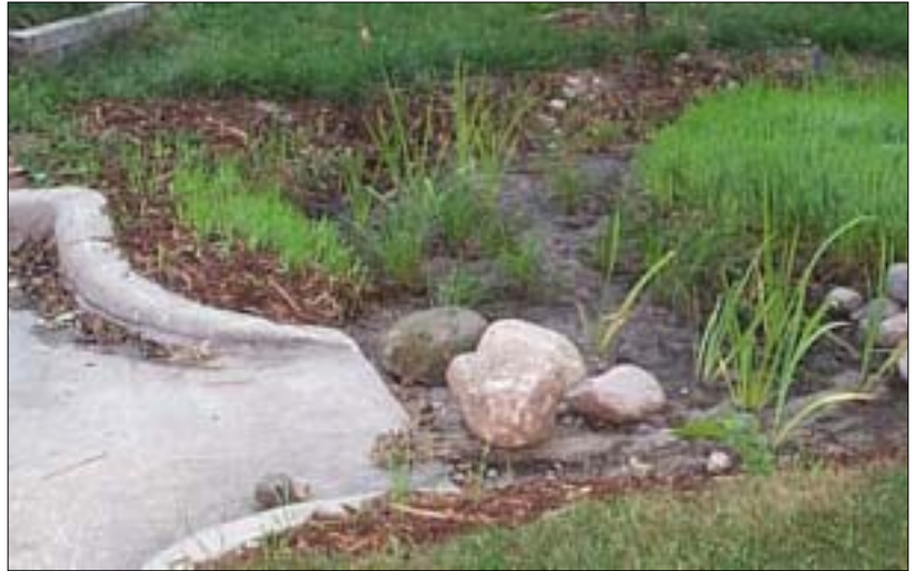
A curb cut into a small bioretention area (Photo: Applied Ecological Service, Inc.)
