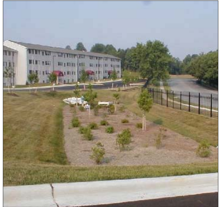
An infiltration basin using bioretention in Largo, Maryland (Photo: Dr. Allen Davis, University of Maryland)
