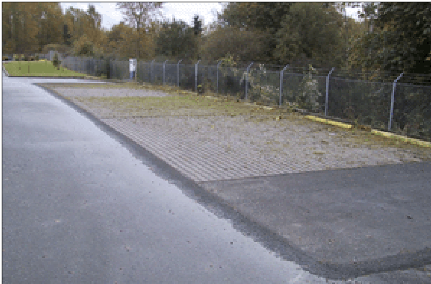
Block Paver and Permeable pavement being tested at the University of Washington (Photo: Center for Water and Watershed Studies)
