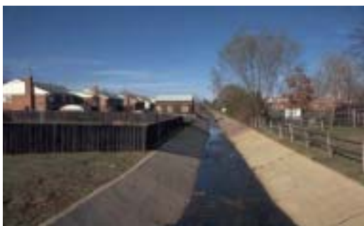
A channelized stream in a suburban neighborhood (Photo: United States Department of Agriculture)
