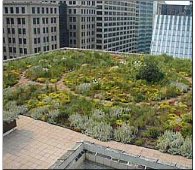
The green roof atop Chicago's City Hall (Photo: Roofscapes, Inc.)
