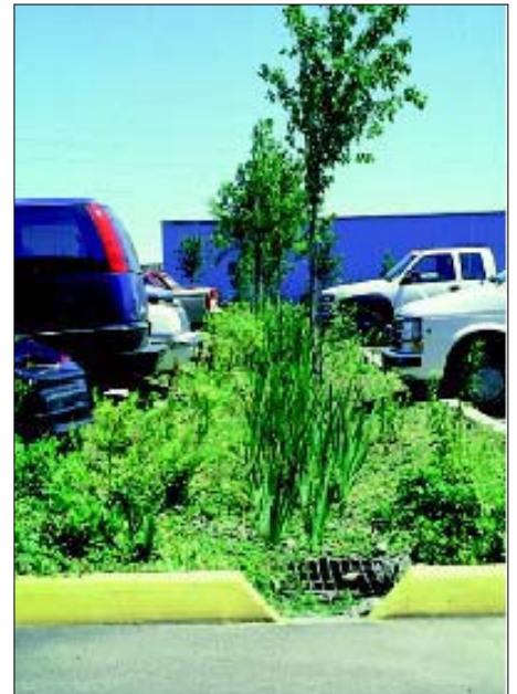
Parking median bioretention with curb cut (Photo: Portland Bureau of Environmental Service)
