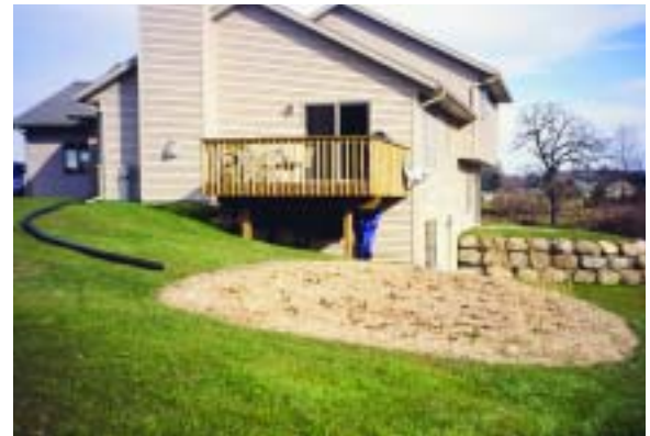
An extension of PVC pipe helps direct downspout water to this rain garden.
