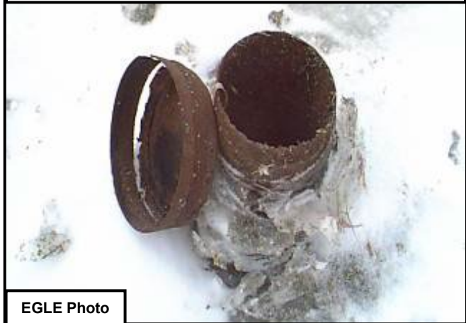
Unsealed abandoned water well that became flooded in Jackson County, Michigan
