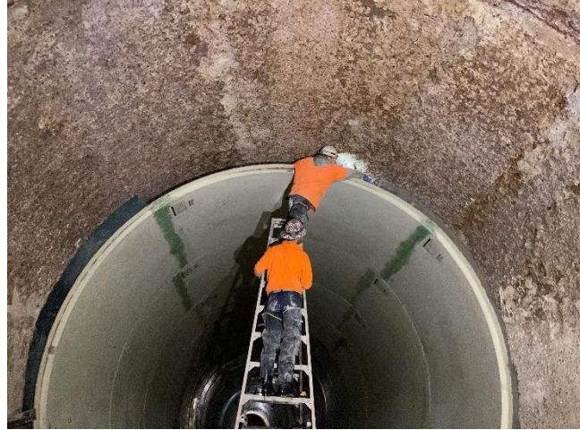
Finalizing bulkhead for grouting efforts
