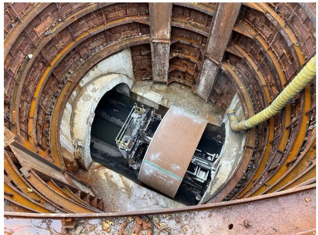
Placing Channeline Segment for Installation
