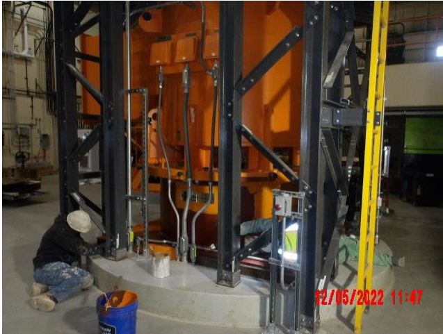
Painting dewatering pumps
