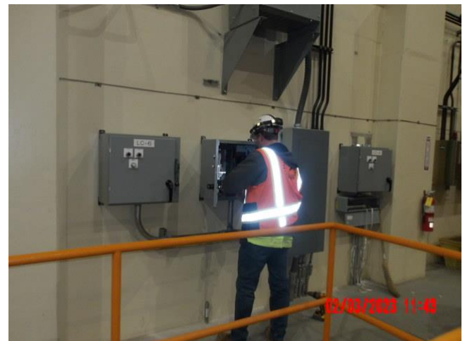
Installation of wet well lighting
