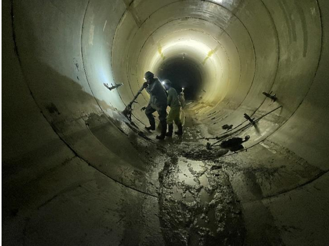
In-sewer grouting activities
