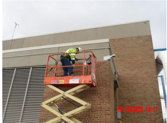
Installing electrical conduit for outside security cameras
