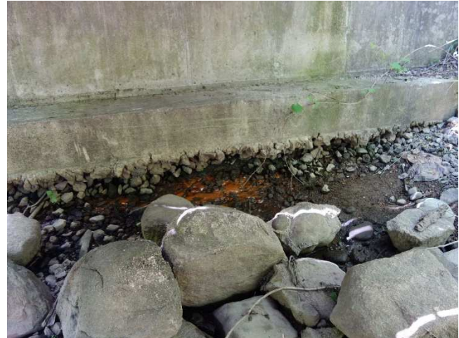
Pictures 25 & 26: Rouge Pedestrian Bridge general condition and south abutment erosion
