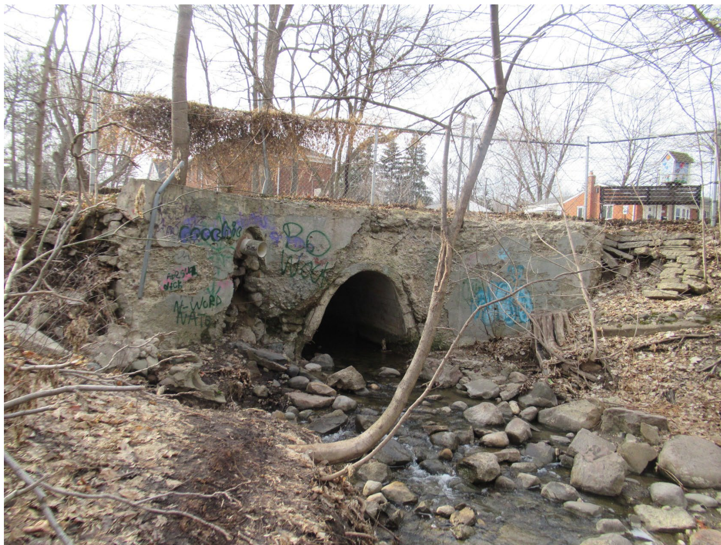
Hutton Street culvert over low flow channel.
