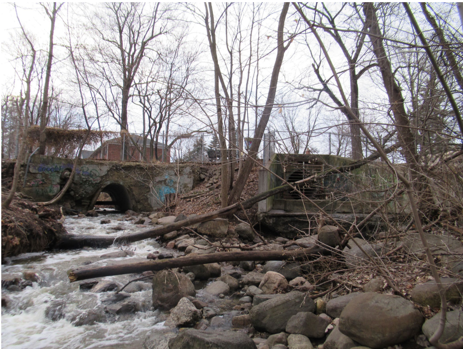
Downstream terminus, looking upstream toward Hutton Street.
