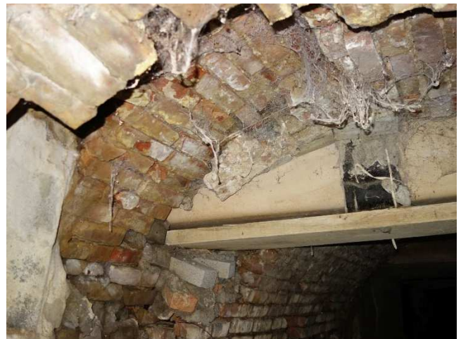
Pictures 15 & 16: Center section (3 and 4) and partial collapse of section 5
