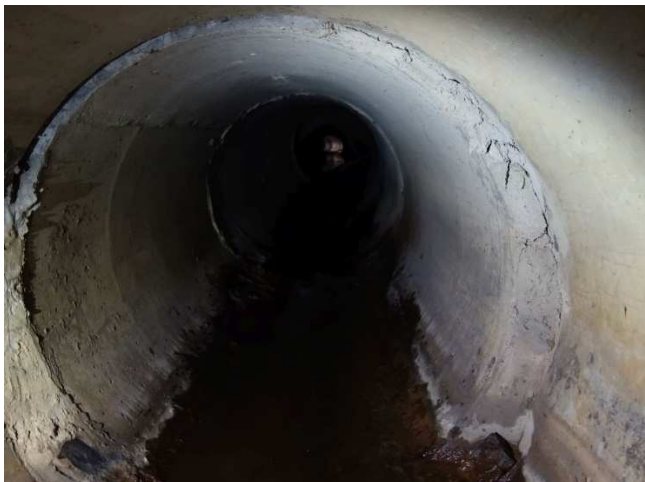
Pictures 15 & 16: Center section (3 and 4) and partial collapse of section 5
