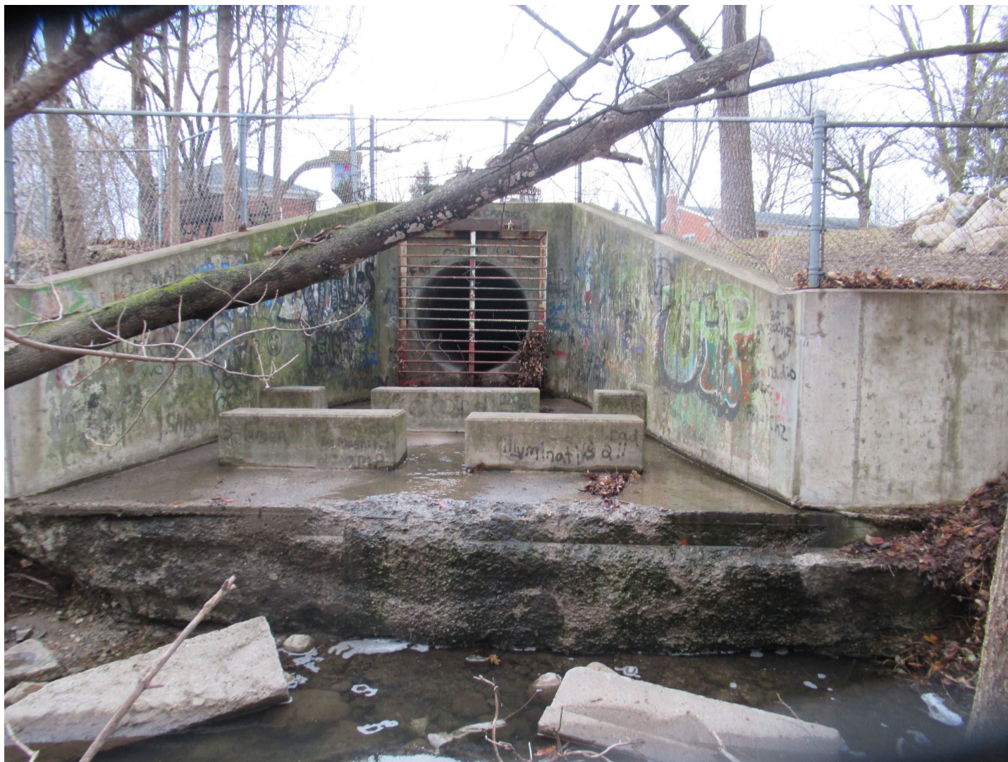
Enclosed portion outlet downstream of Hutton Street.
