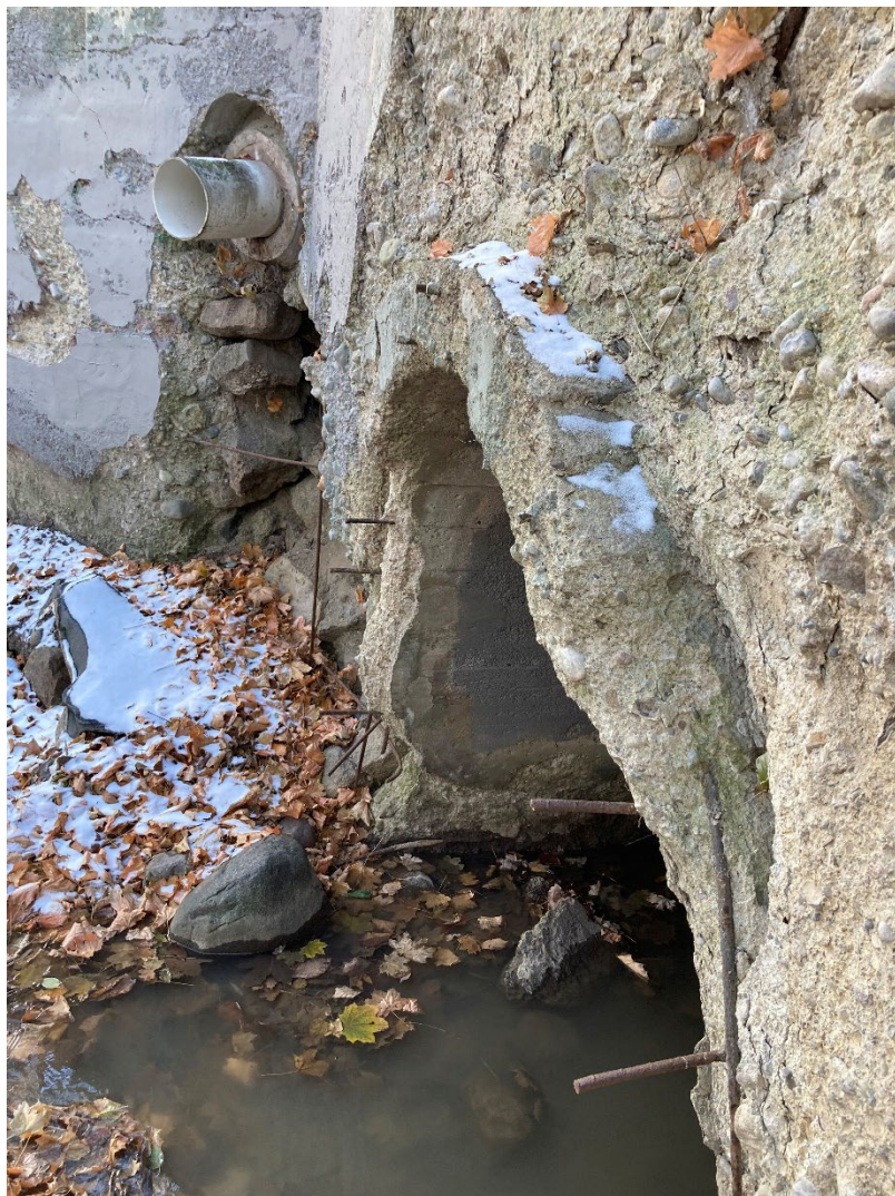
Hutton Street culvert over low flow channel.
