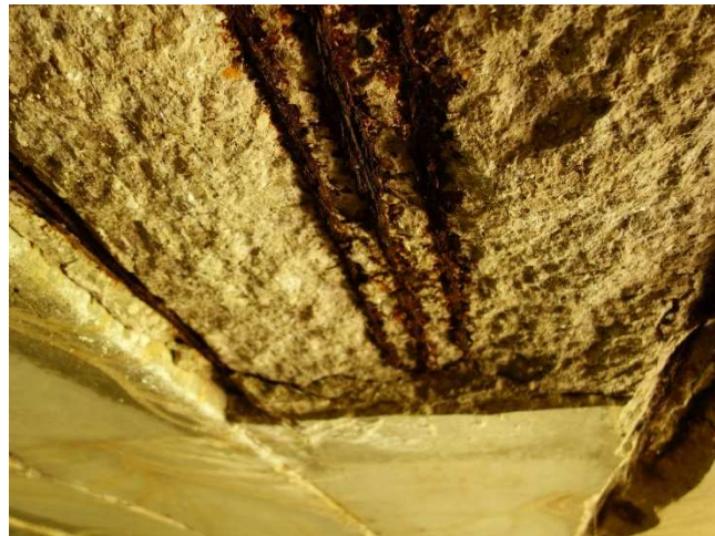
Pictures 11 & 12: Randolph scour hole south abutment and spalling on beams with exposed reinforcement
