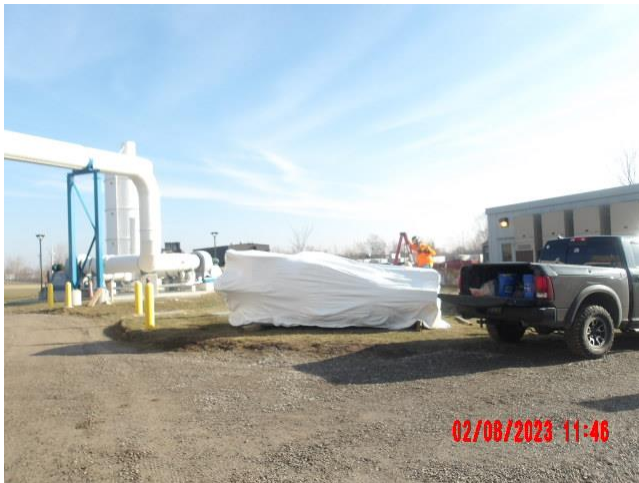
Shrink-wrapping of KGV2 for weather protection
