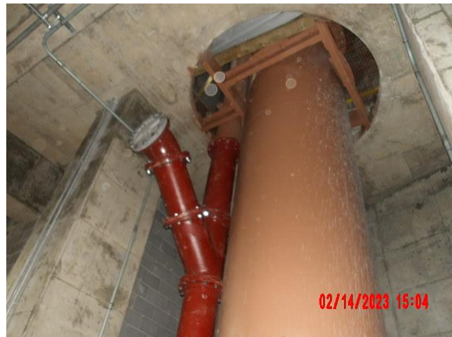
Installation of 12-inch dewatering bypass on fourth floor
