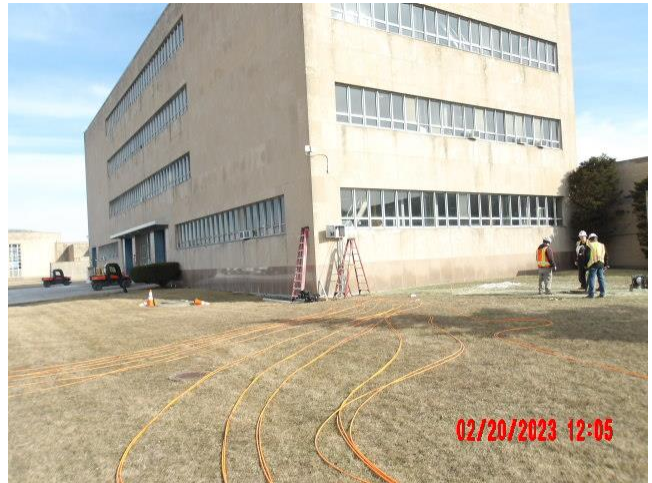
Electrical subcontractor pulling fiber optic cable to NEWTP Chemical Building
