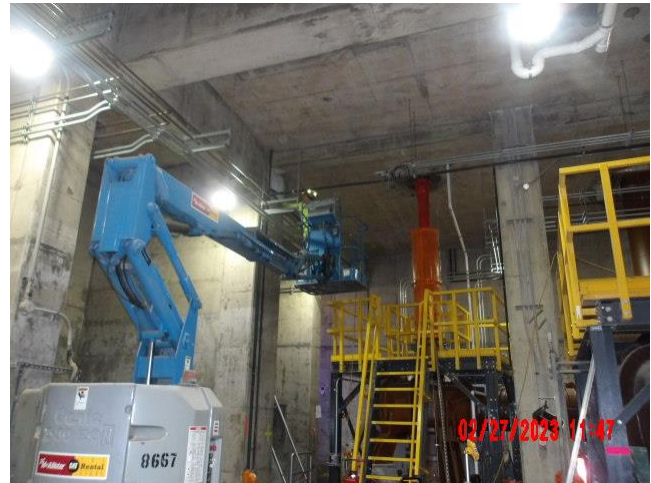
Electrical work on sixth floor
