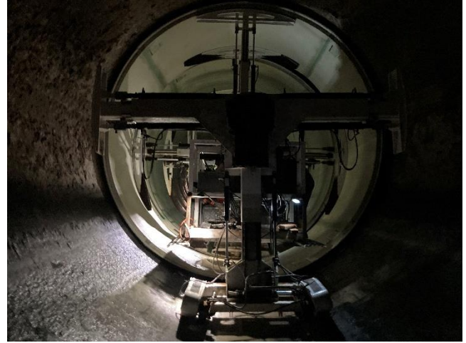
Installation of Channeline pipe sections
