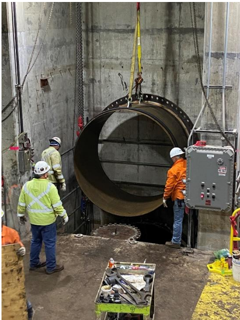
Installation of 84 inch spool as temporary replacement for KGV5
