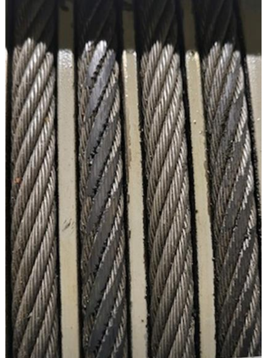
Flat spots observed in dry well elevator support cable
