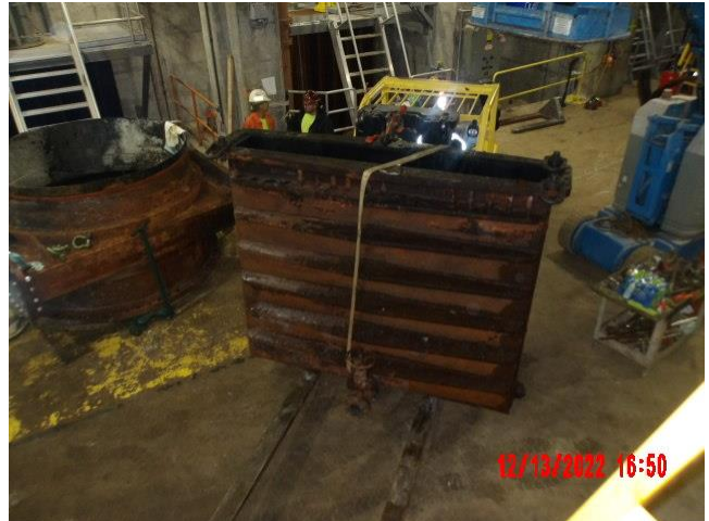
Removed knife (I) and lower part ® from KGV5 on December 12, 2022
