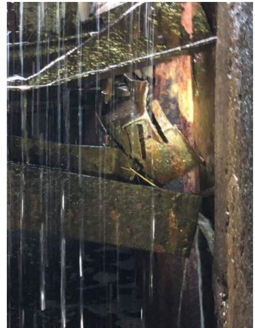
Picture 8: Screen and Strut Structure
