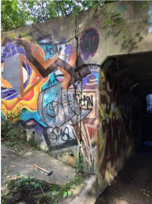
Picture 15: Joint Between Western Retaining Wall and Junction Chamber
