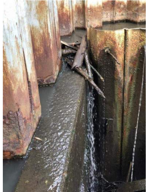
Picture 2: Water Flowing Around Sheet Piling
