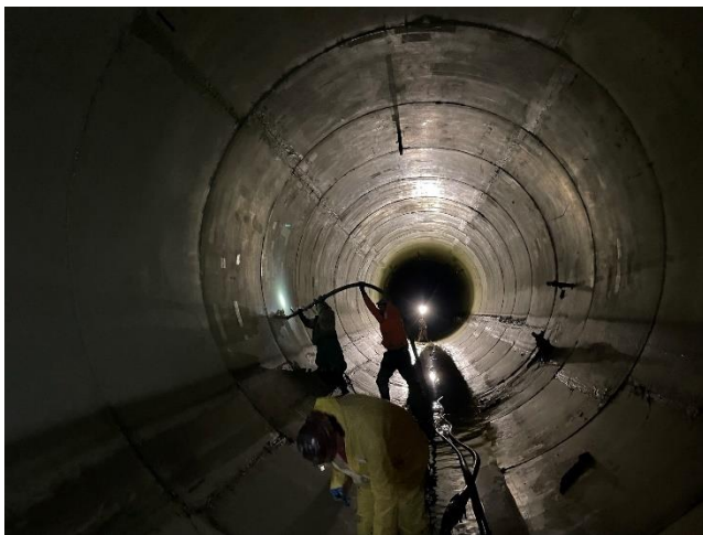
Annular grouting operations
