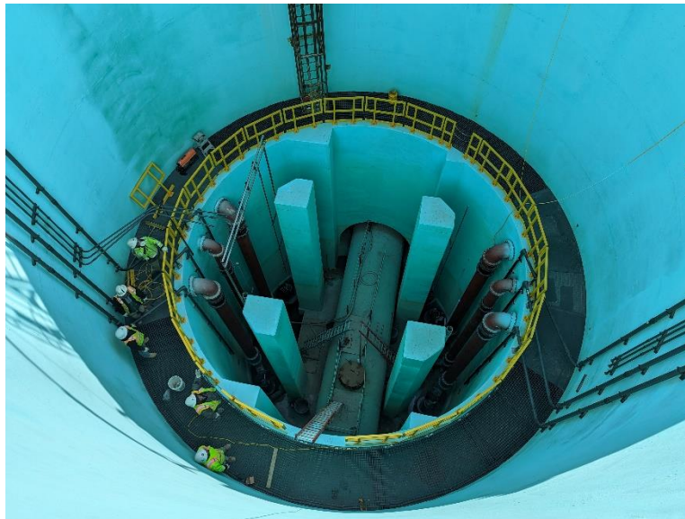
Perimeter flume grating has been installed
