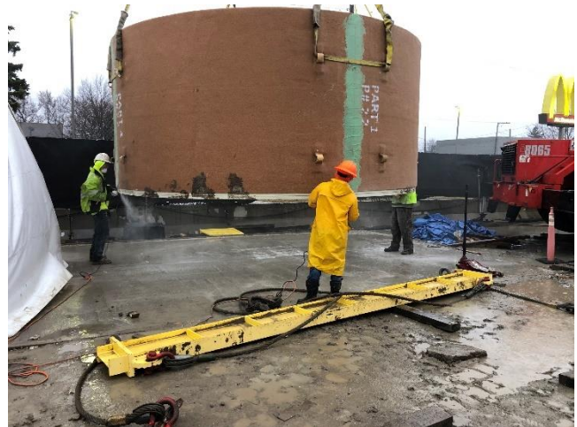
Preparation of spigot prior to installation of Channeline segment
