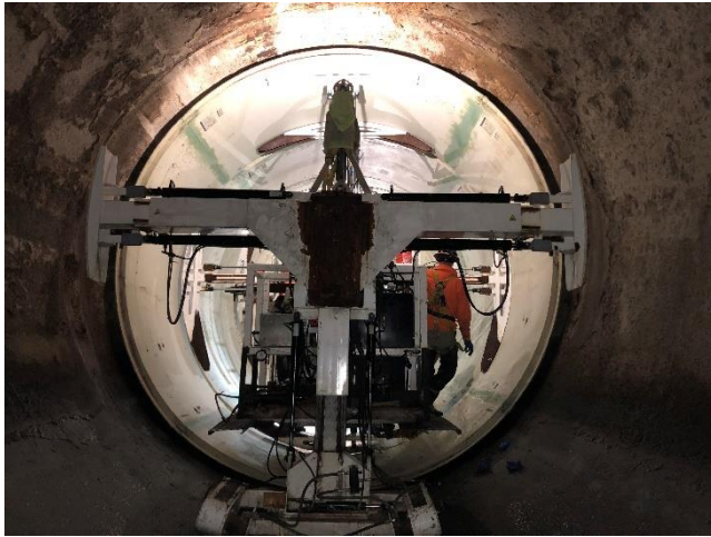
Channeline installation
