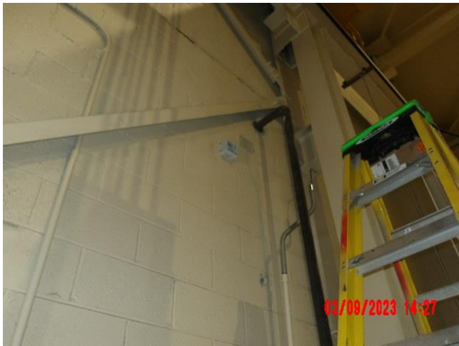
Contractor installing emergency light at Overhead Crane
