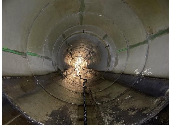
Channeline installation progress
