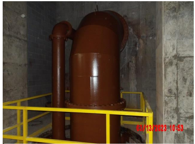
Two coats of paint on Pump #4 discharge pipe
