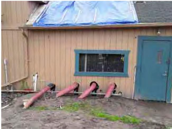
**Inspect ID:** 2022-0020 **Title:** 2704000028\_CELRE\_2022\_A\_2022-0020\_6\_20220506T163908.jpg **Rated Item:** 3. Encroachments **Caption:** Acceptable - An old pump shed noted, sink hole due to corroded pipe underneath. (noted, but not part of project)
