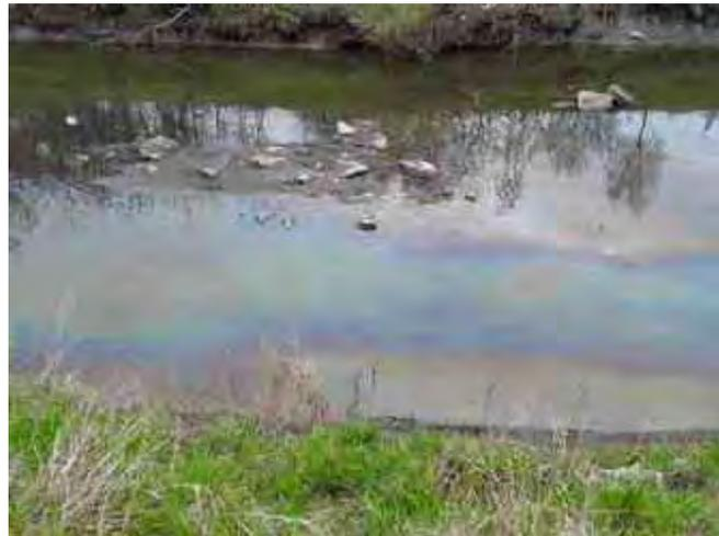
**Inspect ID:** 2022-0023 **Title:** 2704000028\_CELRE\_2022\_A\_2022-0023\_4\_20220506T170628.jpg **Rated Item:** 2. Shoaling (sediment deposition) **Caption:** Minimally Acceptable - Minor shoaling. Noted oily sheen spill. County reported spill, and had oil booms deployed.
