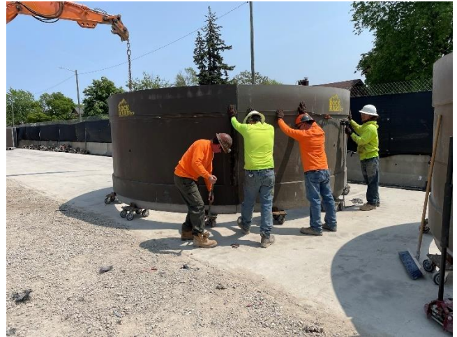
Aligning of Rockhard panels
