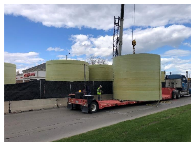
Delivery of QuakeWrap sections
