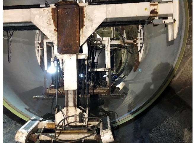
Installation of first QuakeWrap Pipe
