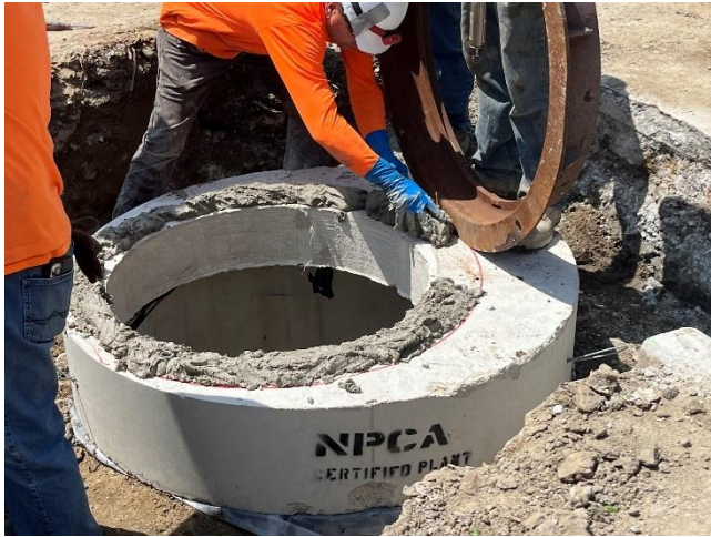
Adjustment to grade of Manhole #104
