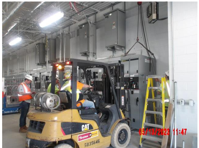
Contractor installing load drop switches (arc flash prevention)
