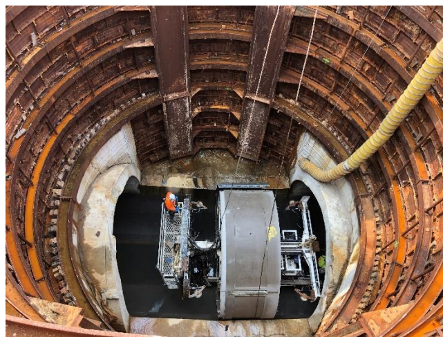
Installation of lining section
