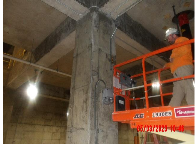
Contractor installing emergency lighting
