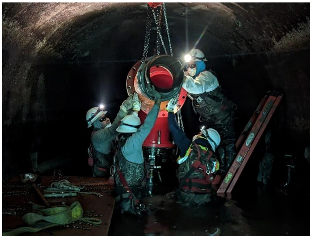
Installation of CS-12 drop pipe
