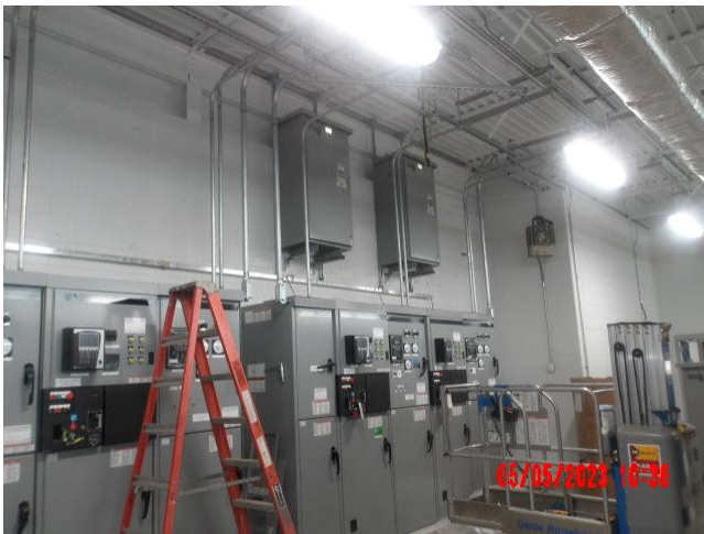
Installation of Pumps transformers
