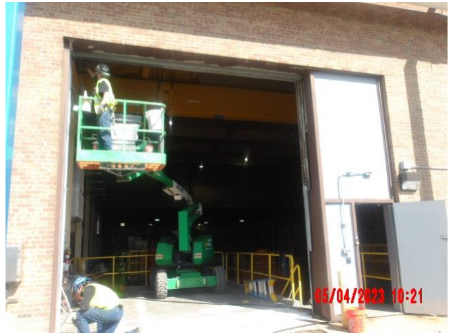
Contractor painting overhead door at locking dock
