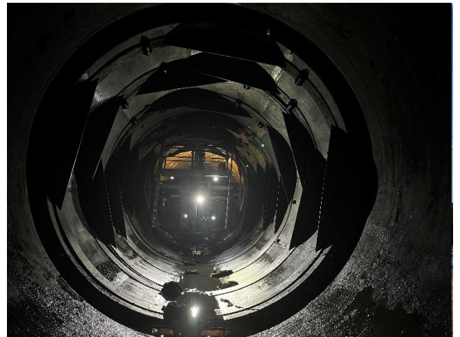
Installation of RockHard pipe section
