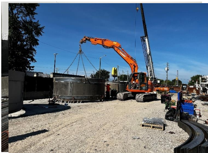
Contractor installing internal bracing
