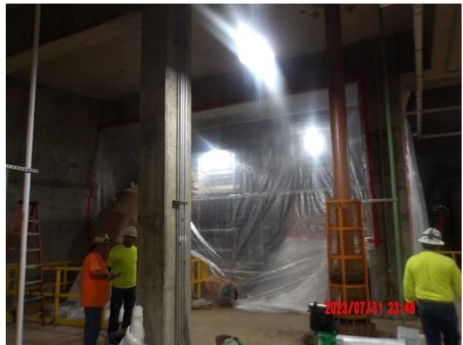
Contractor sandblasting Pump No.2 discharge pipe
