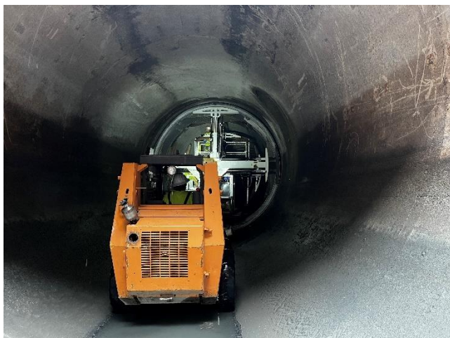
Transporting a RockHard pipe section with skidsteer
