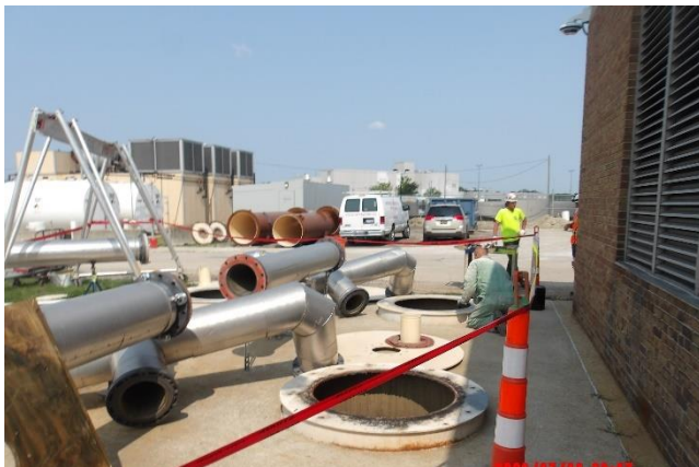
Contractor installing the new gatehouse lid covers
