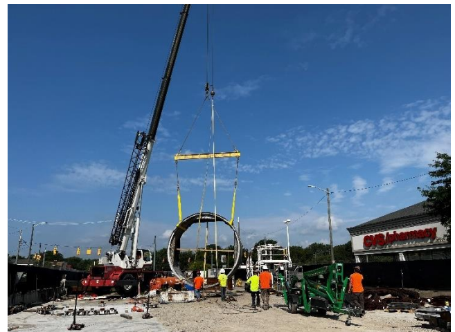
Contractor re-positioning RockHard pipe for installation
