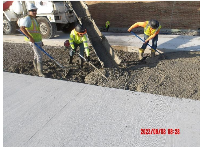
Placement of new subgrade and concrete pavement
