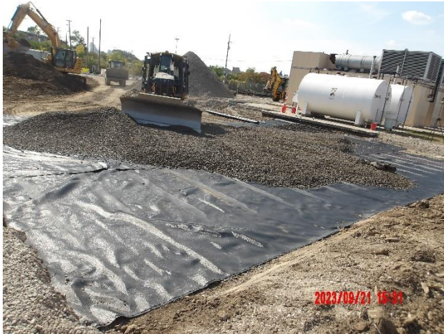
Placement of new subgrade and concrete pavement
