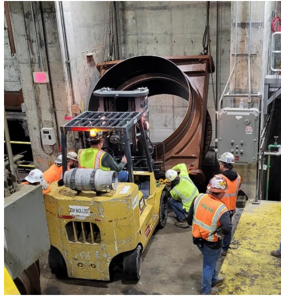
Knife Gate #5 installation
