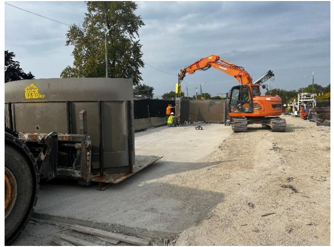
Moving and assembling RockHard panels
