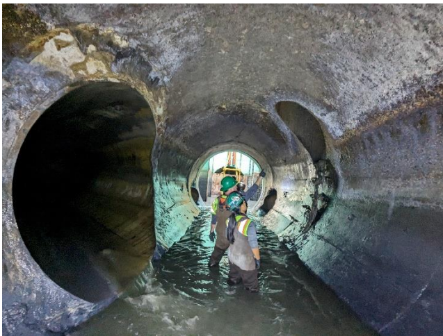
Engineering team inspecting interceptor near CS-12
