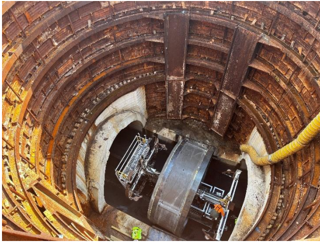
Installation of pipe section P#9
