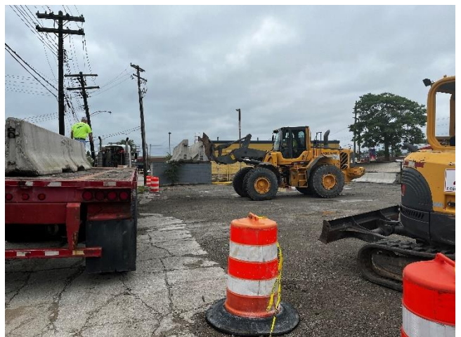
Placing jersey barrier
