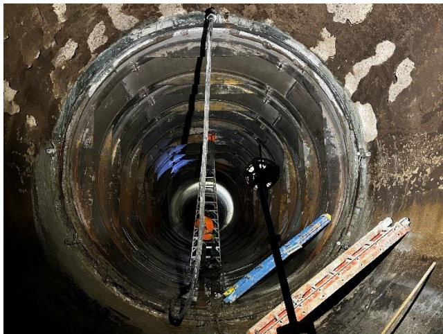
Grouting third lift through manhole MH105
