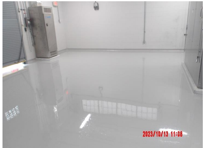
Final epoxy coat at new electrical building
