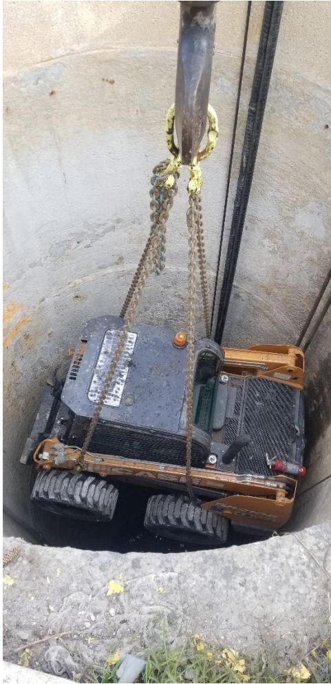
Lowering debris removal equipment into MH-12A-5
