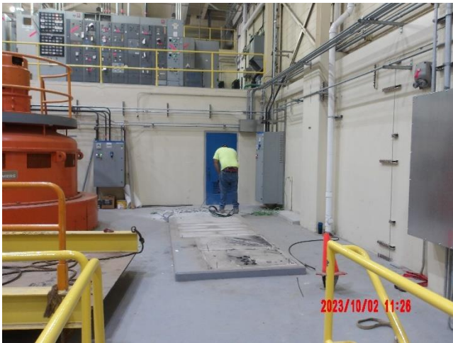
Contractor demolishing P4 panel footing
