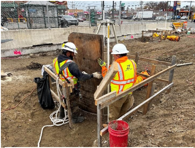
Contractor lowering in formwork for bulkhead
