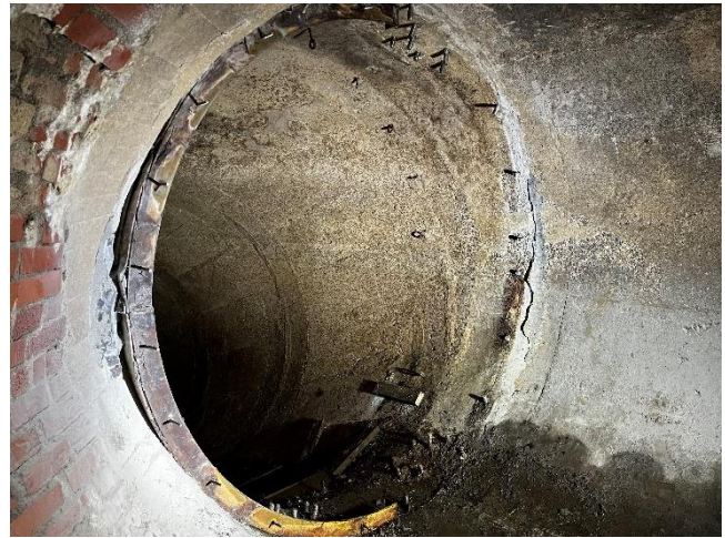
Connection of 8' sewer to PCI-4
