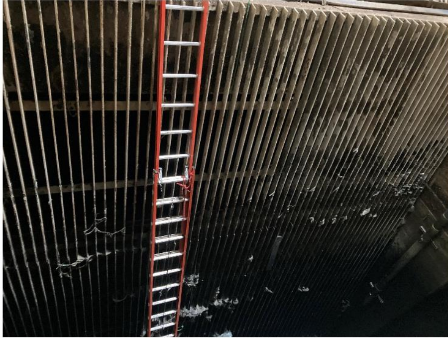
Lakeshore Chamber Bar Screen
