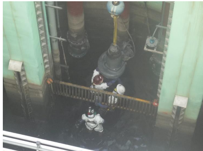
Contractor working on CS-12 pumps.
