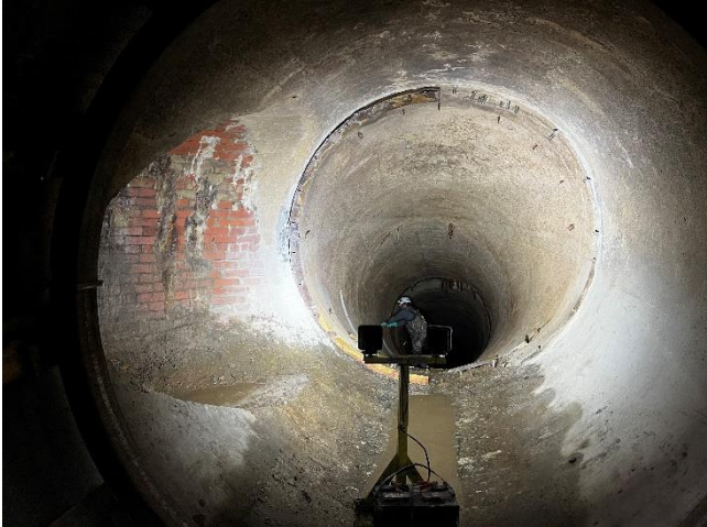
Preparation for formwork between 8' sewer and PCI-4
