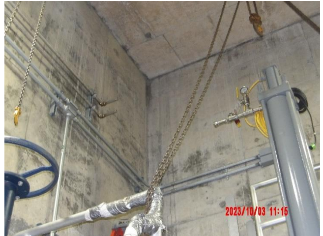
Installation of Pump #5 actuator
