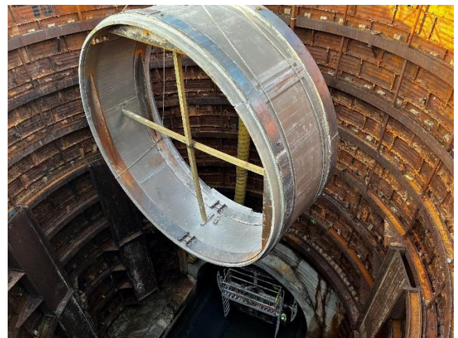
Lowering RockHard pip section into shaft for installation
