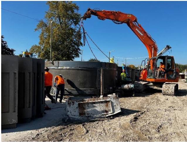
Ongoing assembly and bracing of RockHard pipe sections
