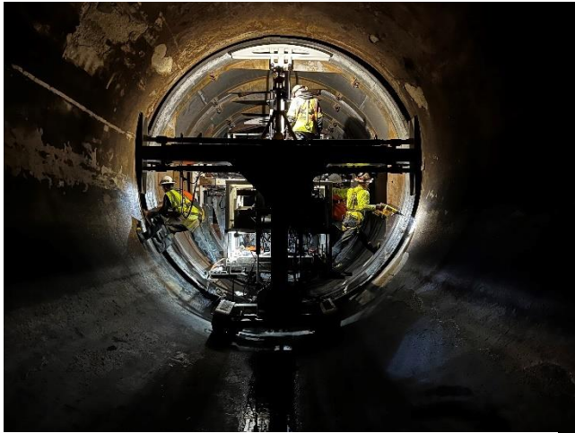
Installation of RockHard pipe section
