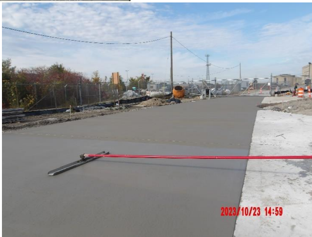
Contractor pouring Phase II concrete
