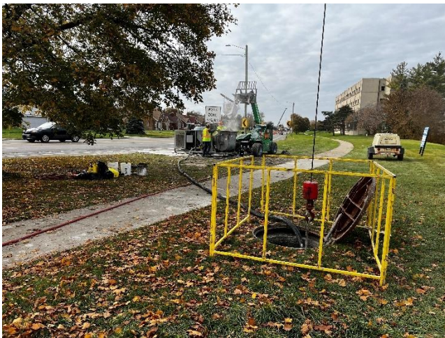
Contractor pouring Quadflow for lining transition section
