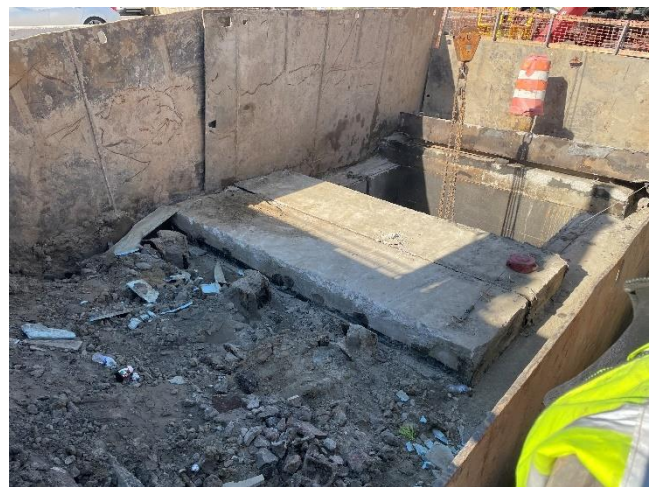
Removal of PC 663 precast cover
