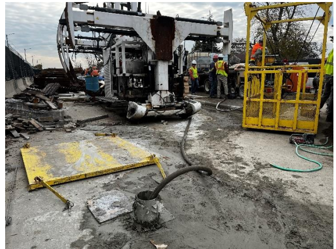
Subcontractor filling dewatering wells at Access Shaft
