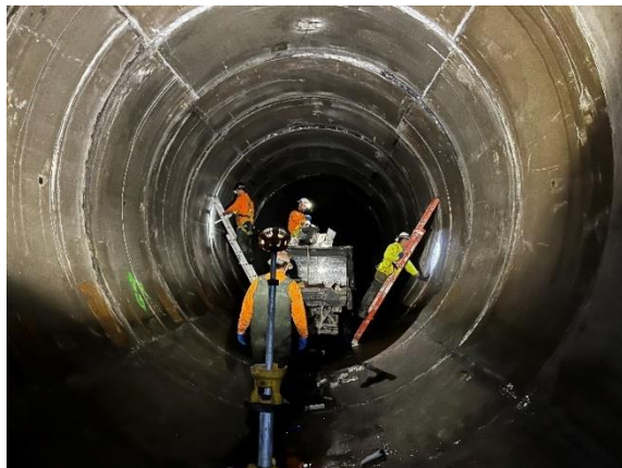
Contractor smoothing RockHard joints
