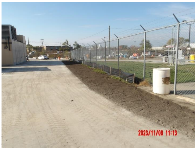
Placement of topsoil behind concrete
