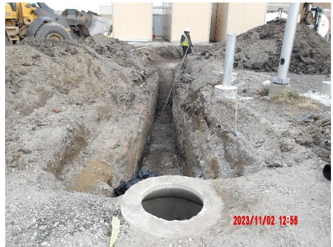
Installation of 6 inch edge drain
