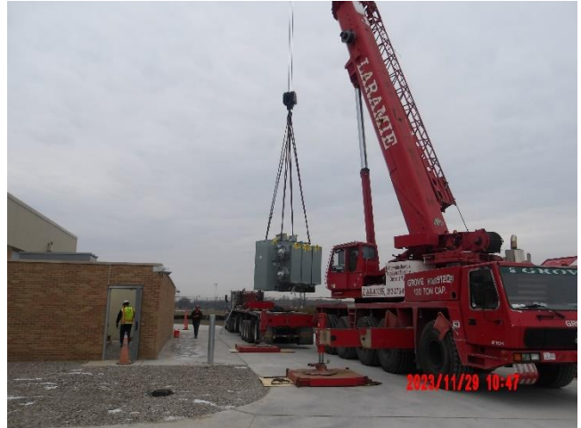
Delivery of Transformer #4 by Laramie Crane
