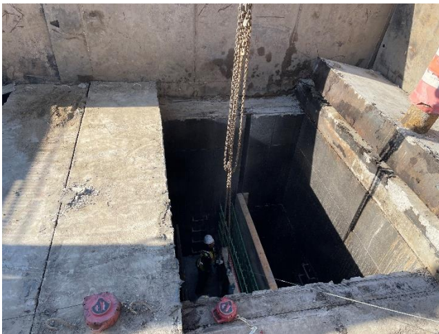
Removal of PC 663 precast cover
