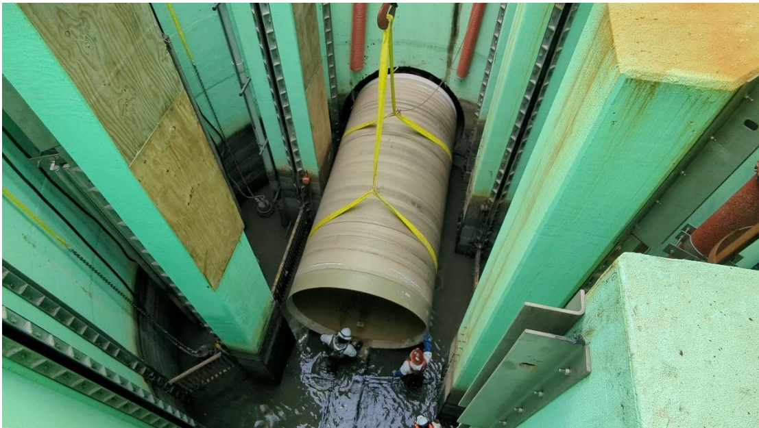
Lining from Control Structure 12
