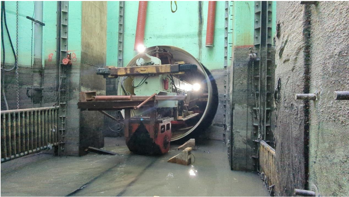
Lining from Control Structure 12
