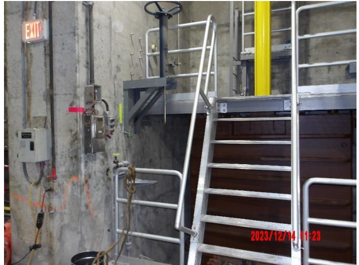
Installation of 6-inch knife gate valve at KGV3
