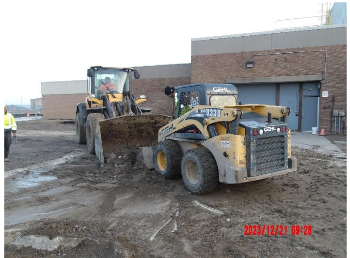
Removing contaminated soil to special dumpster
