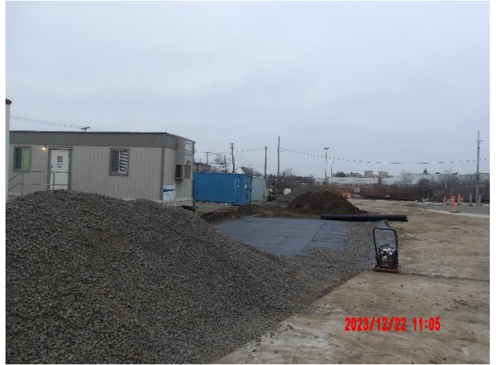
Removing surficial soils to and placing geotextile and 21AA limestone
