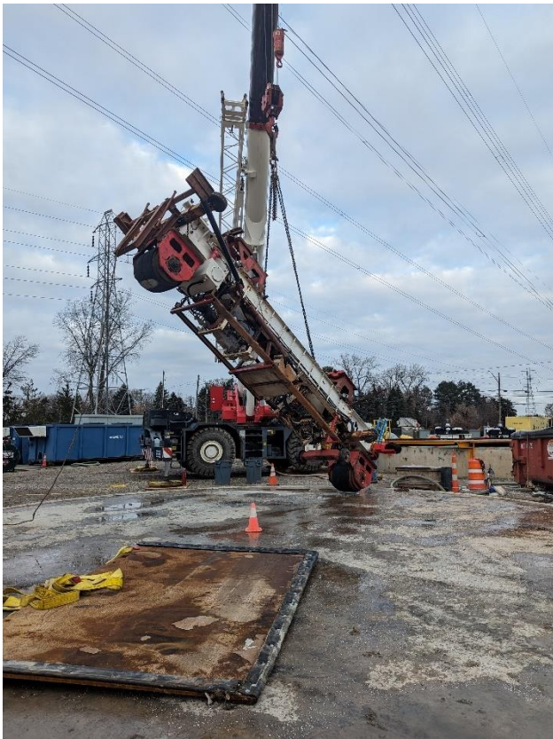
Staging the pipe carrier
