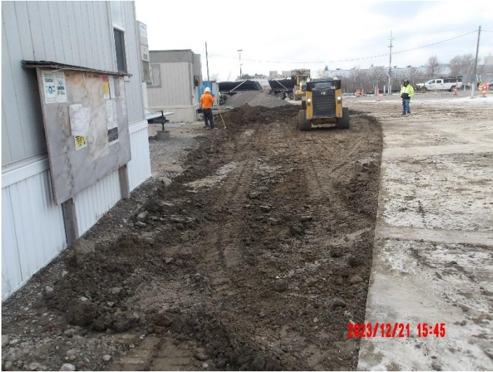
Removing surficial soils to and placing geotextile and 21AA limestone
