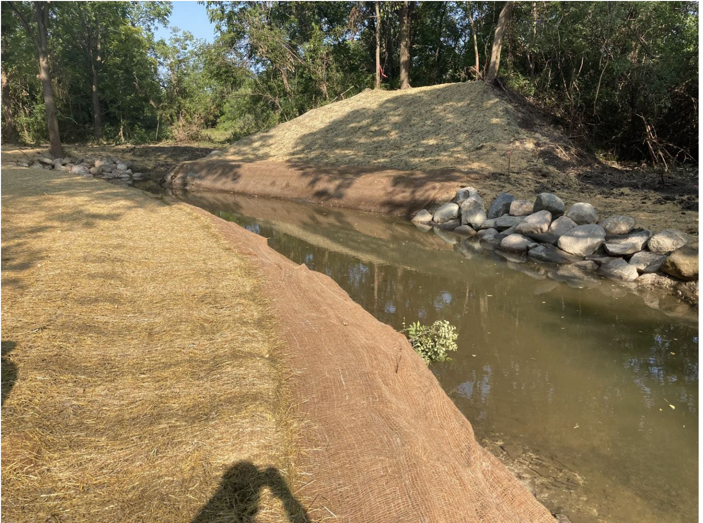
Photo 3 – New channel through rail siding crossing
