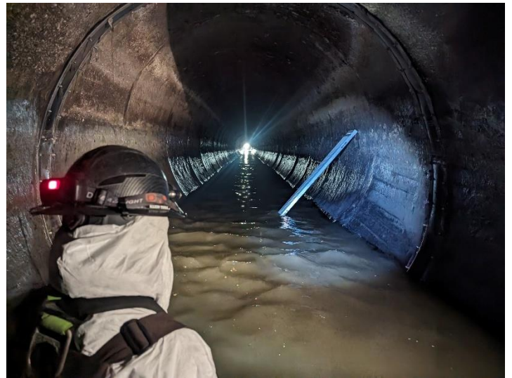
In pipe during lining operations
