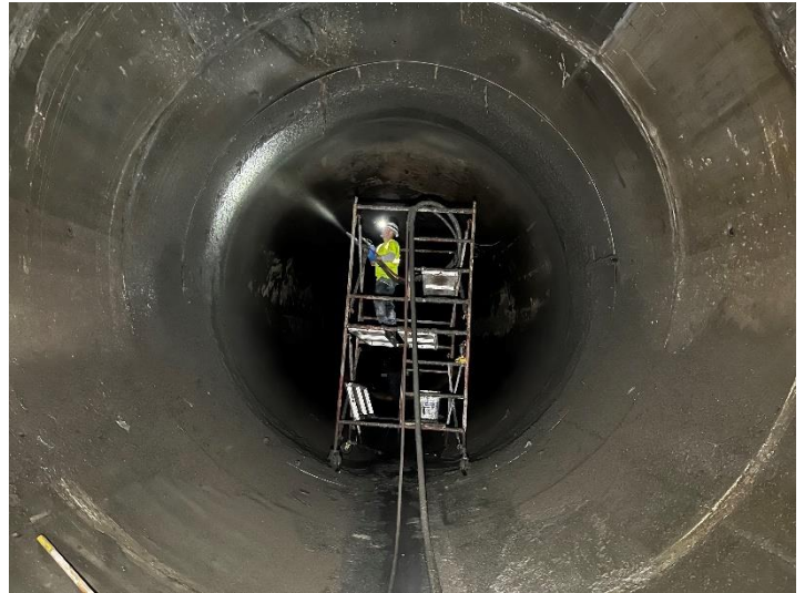
Application of shotcrete to RockHard transition section
