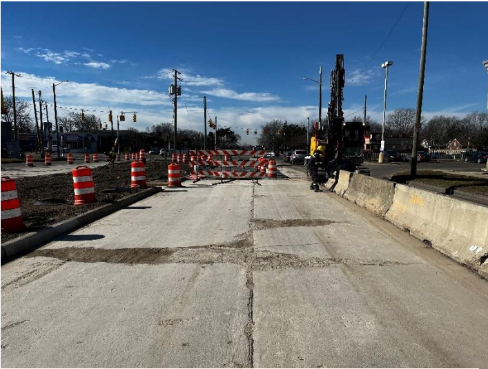
Replacing concrete jersey barrier with traffic cones and Type IIIs
