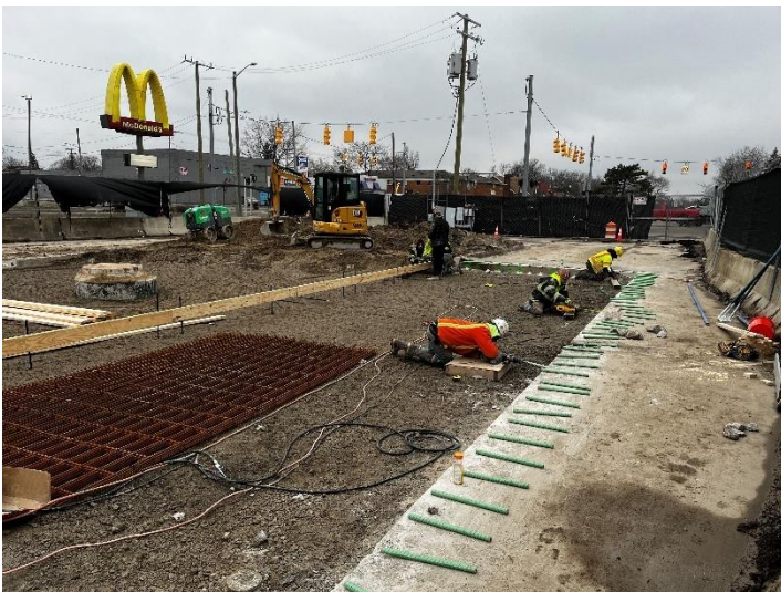
Preparing for pavement replacement
