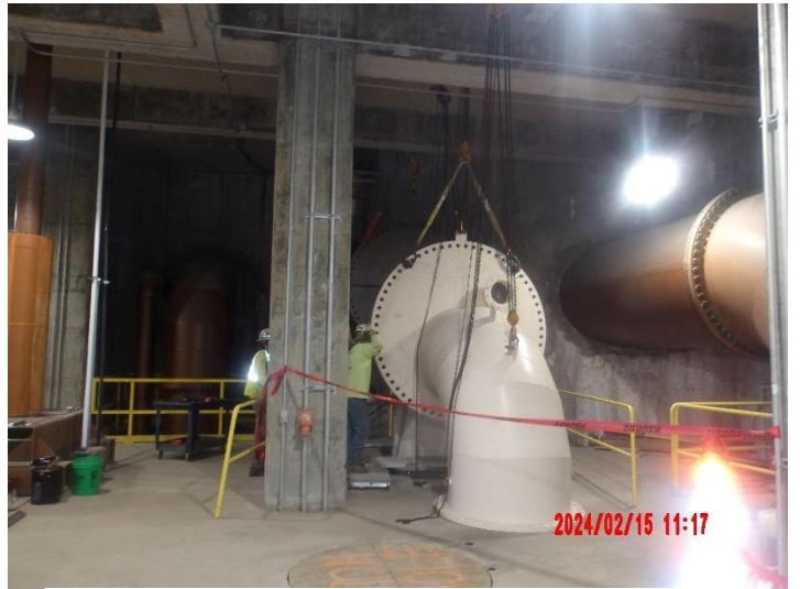
Installing 90° elbow at Pump #5
