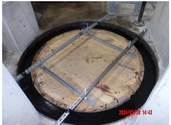
Preparing to pour the DEVCON gasket for the Pump #5 suction spool
