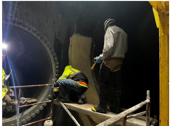
Armoring the transition of the discharge chamber
