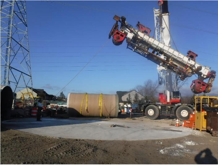
Positioning pipe carrier for lining operations
