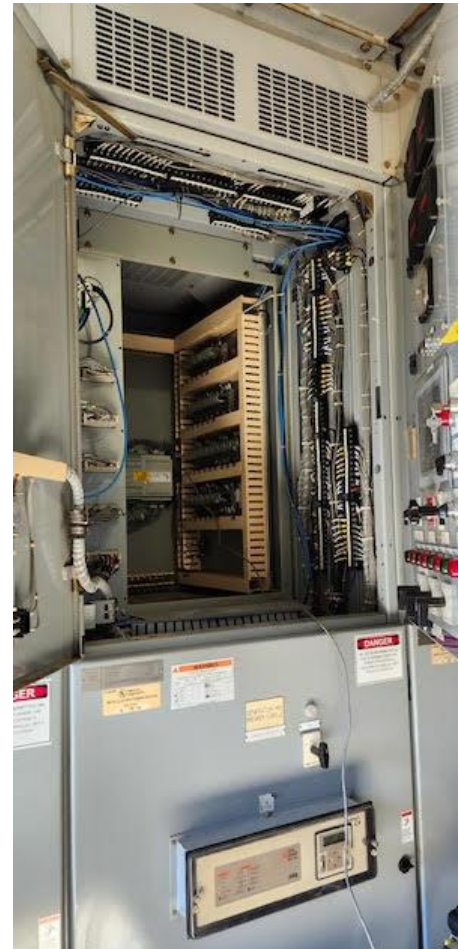
Finishing DSLC-2/MSLC-2 Upgrade
