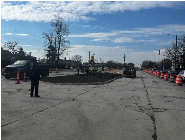
Restoration of Outer Drive median
