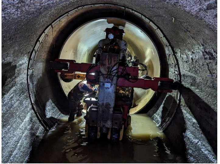
Positioning pipe carrier for lining operations
