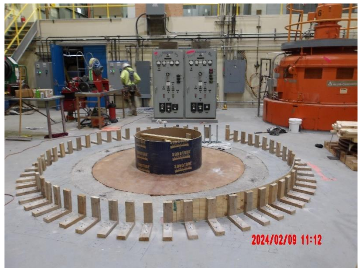
Construction of Pump #5 concrete footing
