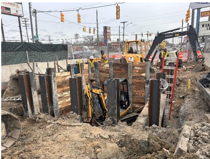
Progress on Temporary Earth Retention System
