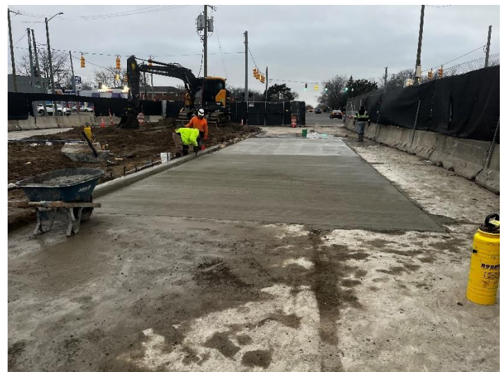
Finishing pavement replacement
