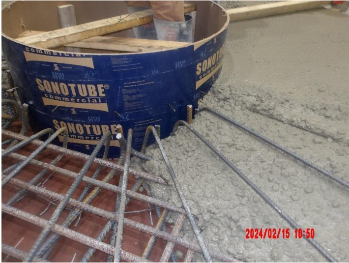
Concrete placement for Pump #5 footing
