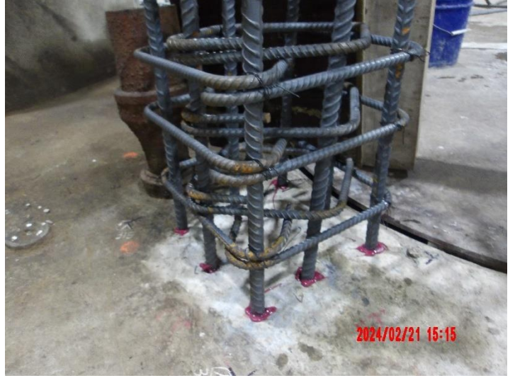
Assembly of Pump #5 pedestal reinforcement
