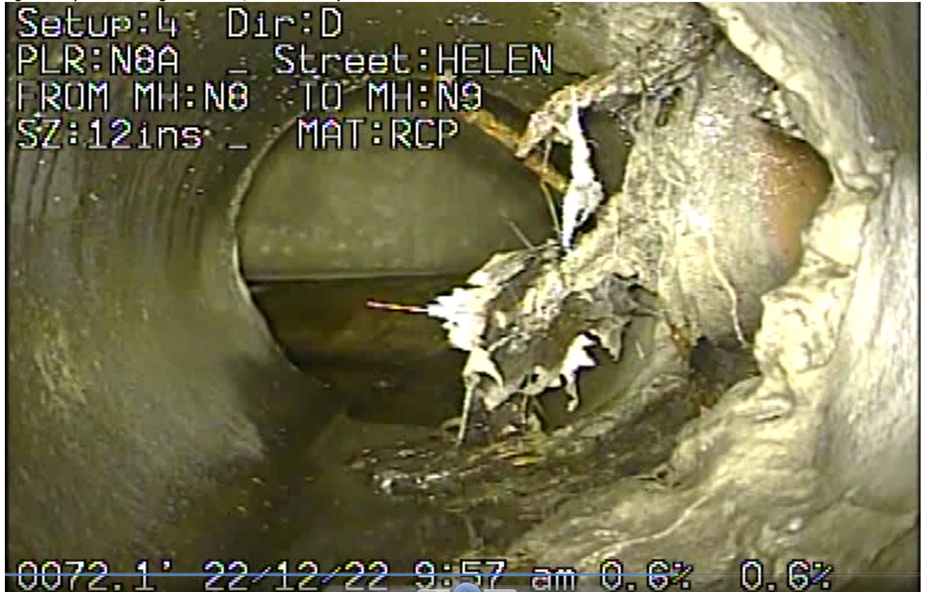
Figure 2. Tap in drain along Helen Street, south of Cherry Hill Road
