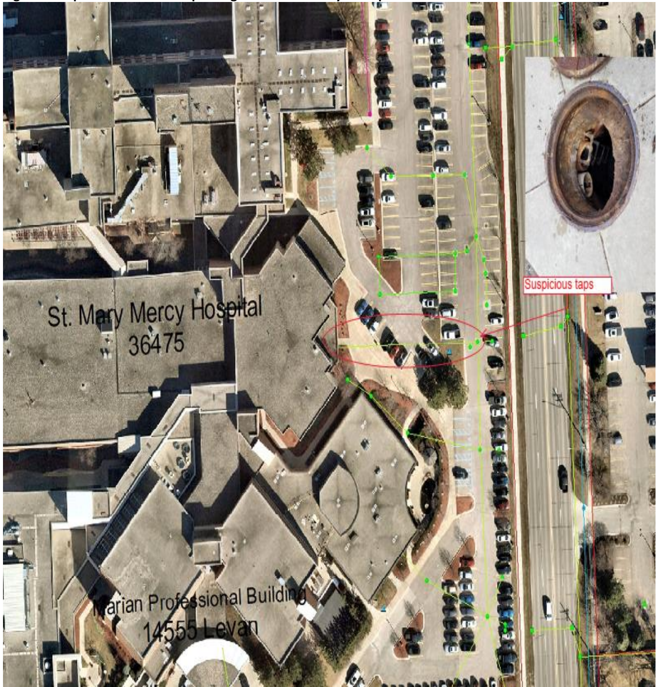
Figure 2. Tap to Storm Drain in parking lot of Saint Mary's Hospital
