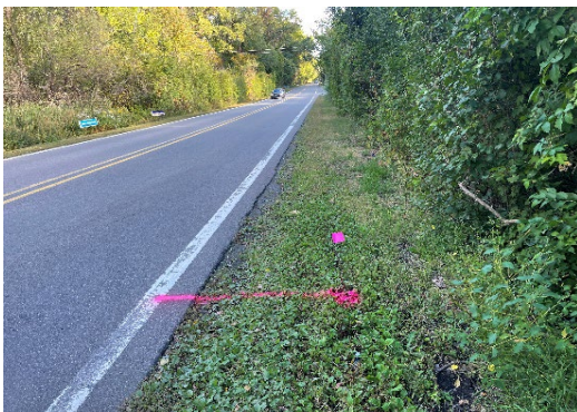
Sign installation location marked with pink paint and flag
