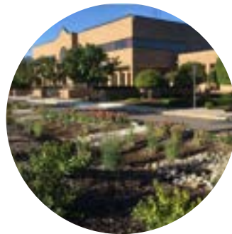
Bioswale installation at Clinton Township Civic Center
