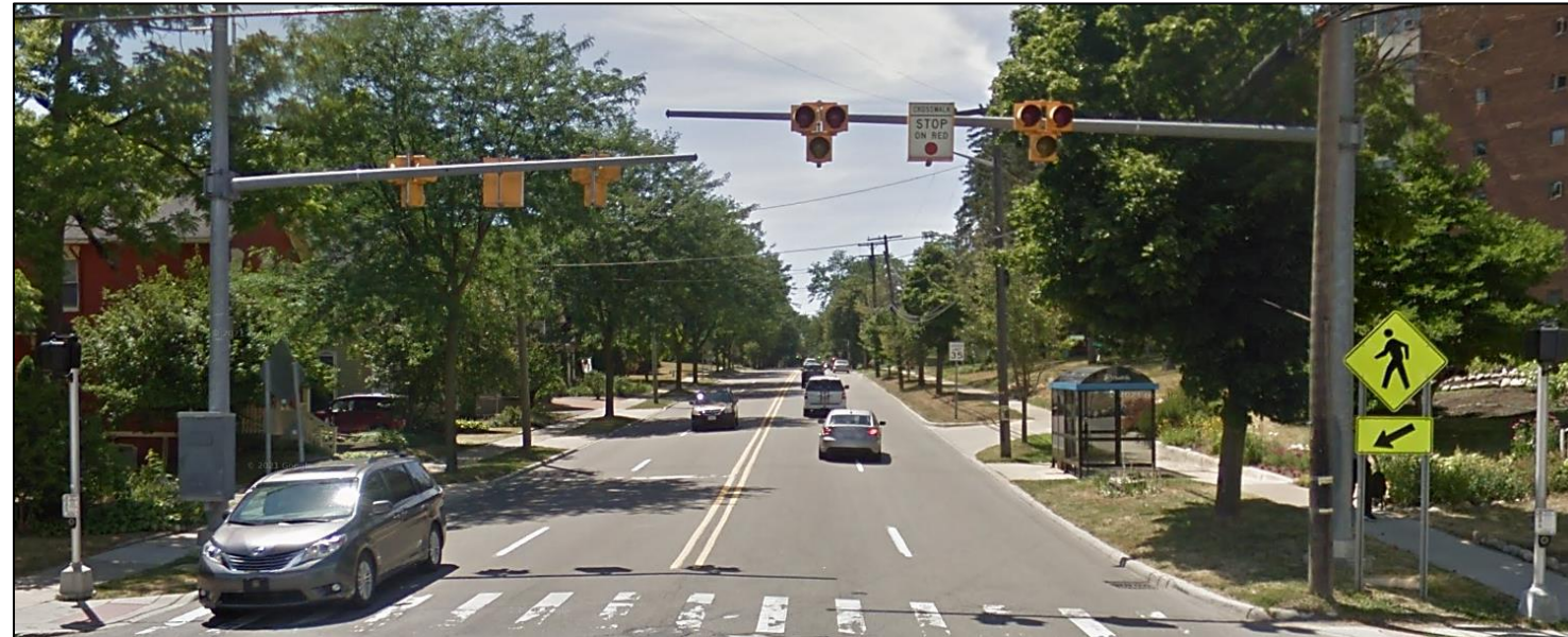
Image: PHB Pedestrian crossing near bus stop on Huron St in Ann Arbor
