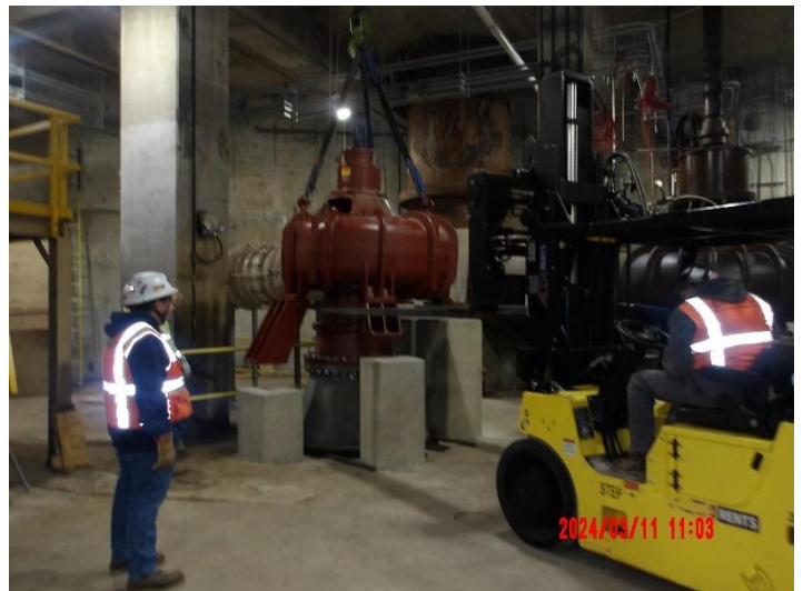
Installation of Pump #5 on sixth floor
