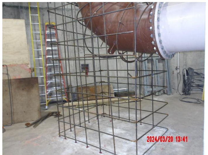
Building the Pump #5 thrust block
