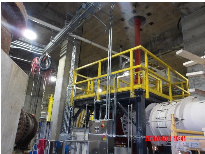
Installing Pump #5 seal and electrical conduits
