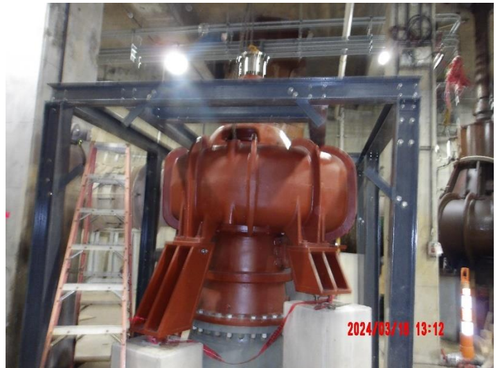
Installing Pump #5 platform
