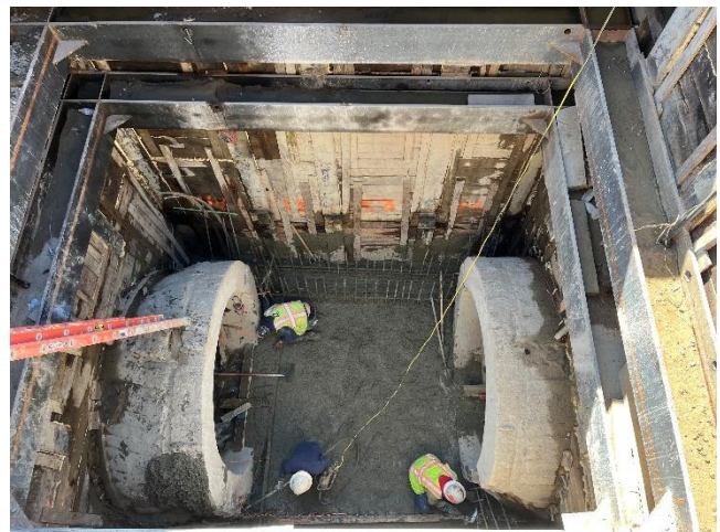
Placement of structural base slab at PC-663
