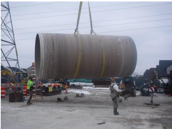
Lowering Hobas pipe into CS-12
