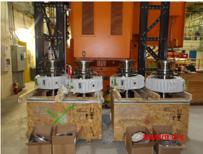
Installing Pump #5 shaft bearings
