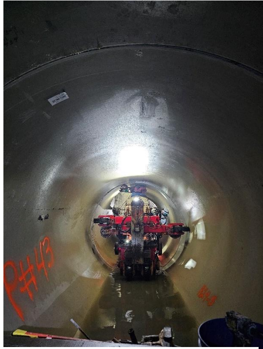
Installing Hobas pipe section with pipe carrier
