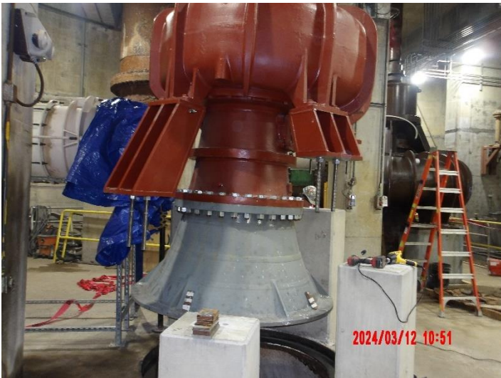
Construction Anchoring and adjusting Pump #5
