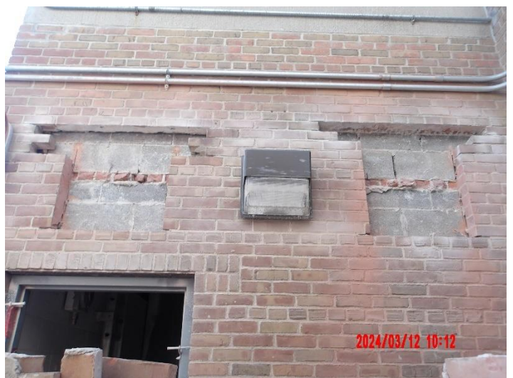
Construction of mechanical openings at wet well elevator
