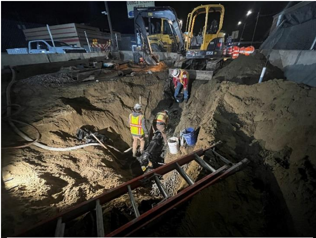
Water main relocation near 7 Mile gate structure
