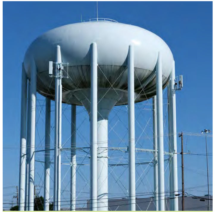
Water Tower, City of Pontiac
