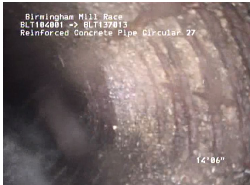
Exposed Reinforcement
