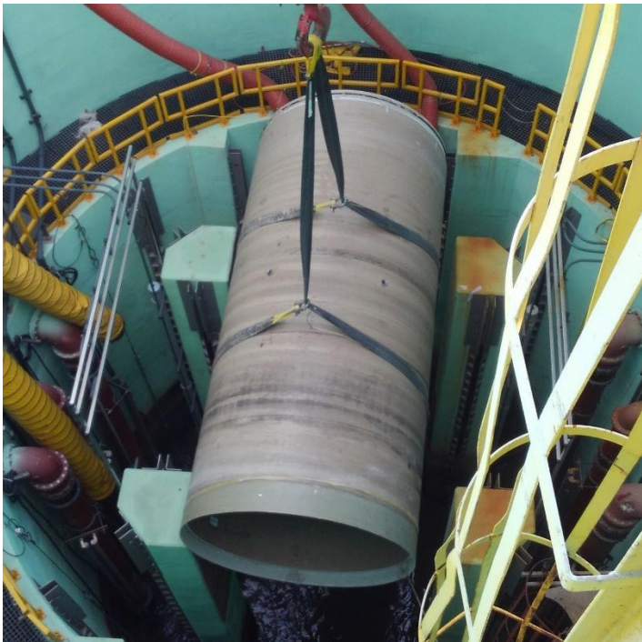
Contractor lowering Hobas pipe segment into CS-12
