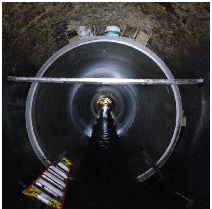
View of lined pipe section
