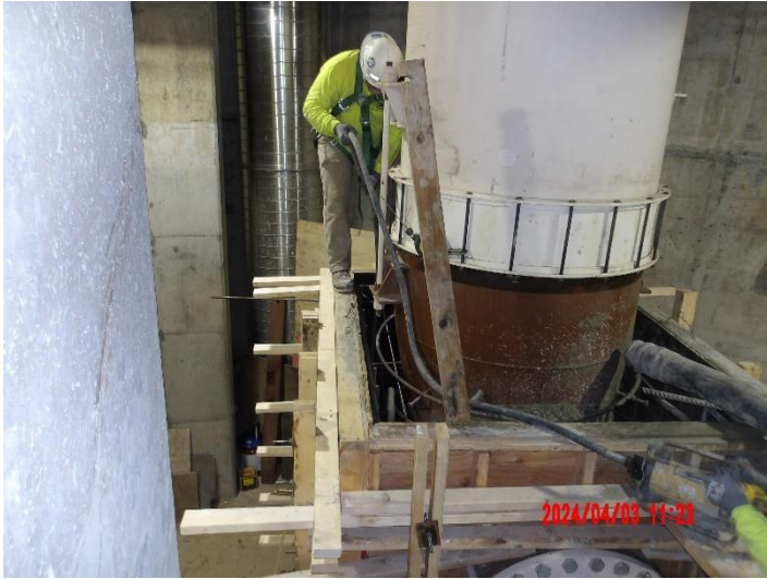
Contractor placing concrete for Pump #5 thrust block
