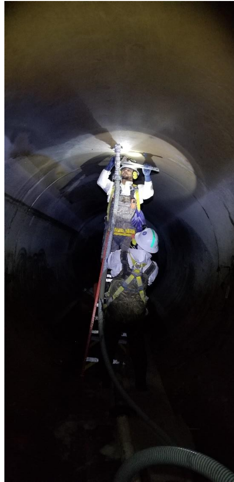
Contractor performing annular grouting
