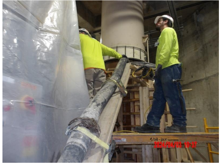
Contractor placing concrete for Pump #5 thrust block
