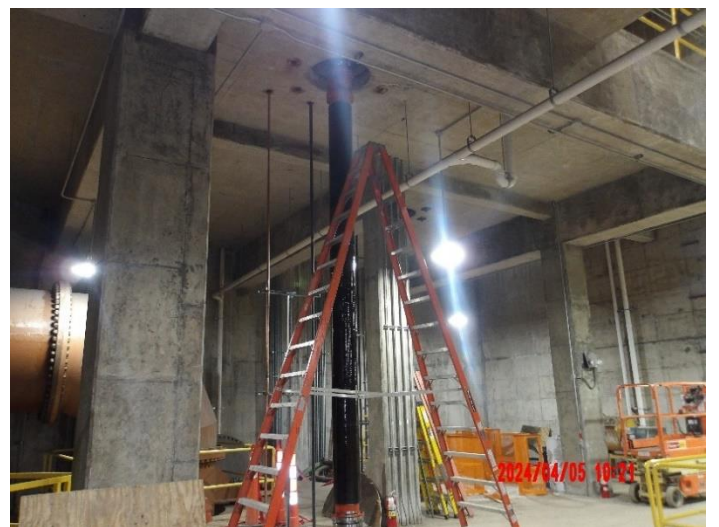
Aligning Pump #5 shaft on third floor
