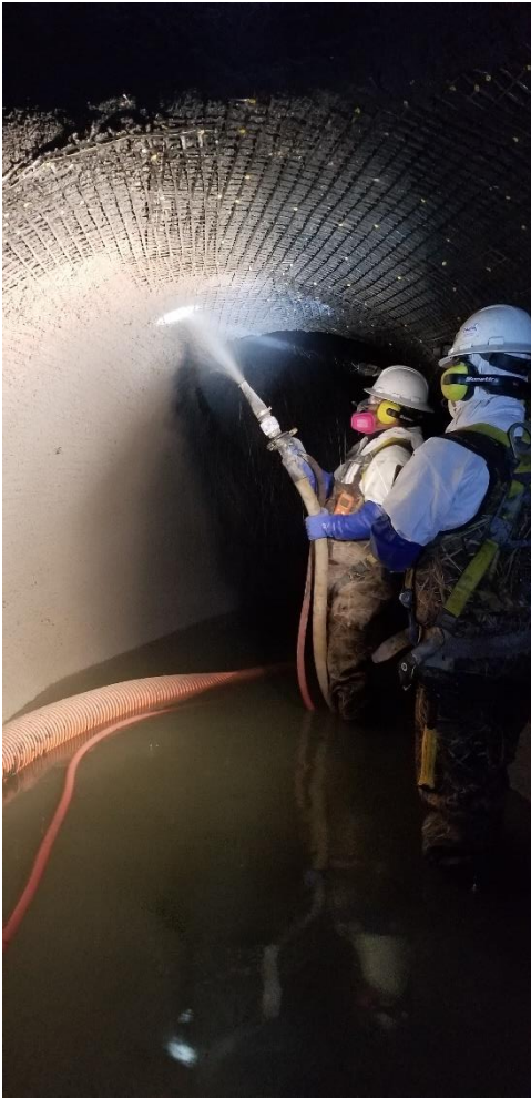
Contractor preparing for spray lining in the 8 foot section
