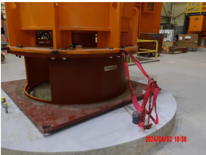
Installation of Pump #5 electric motor and stand
