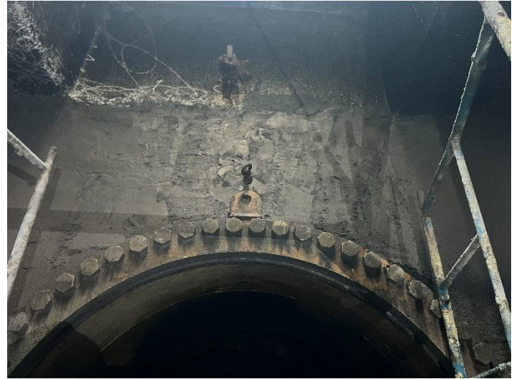
Cementitious lining on drop beam adjacent areas
