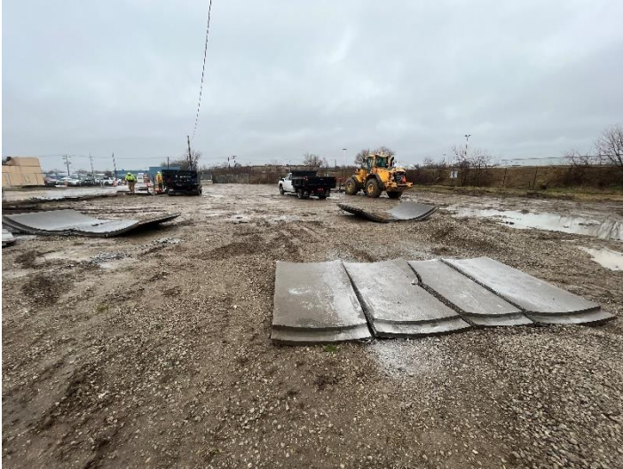
Contractor removing RockHard panels from laydown area
