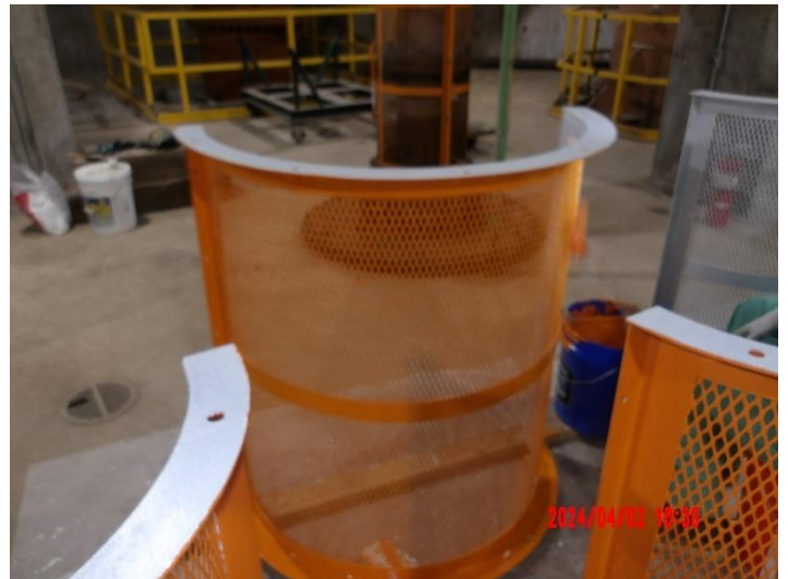
Painting shaft guards for Pump #5
