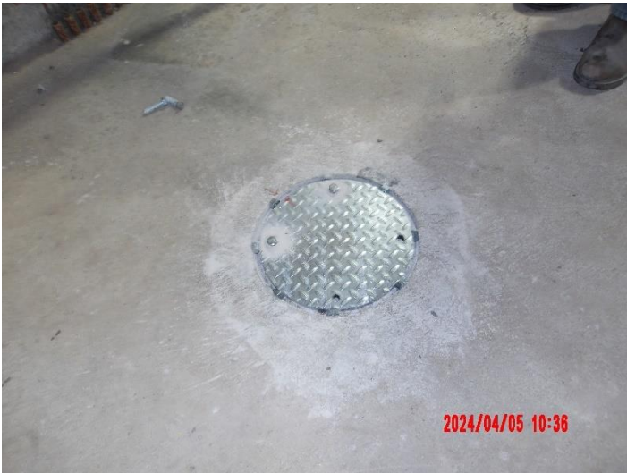
New metal plate covering of KGV access openings on fifth floor
