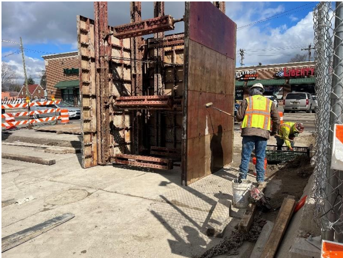
Contractor applying release agent to concrete formwork
