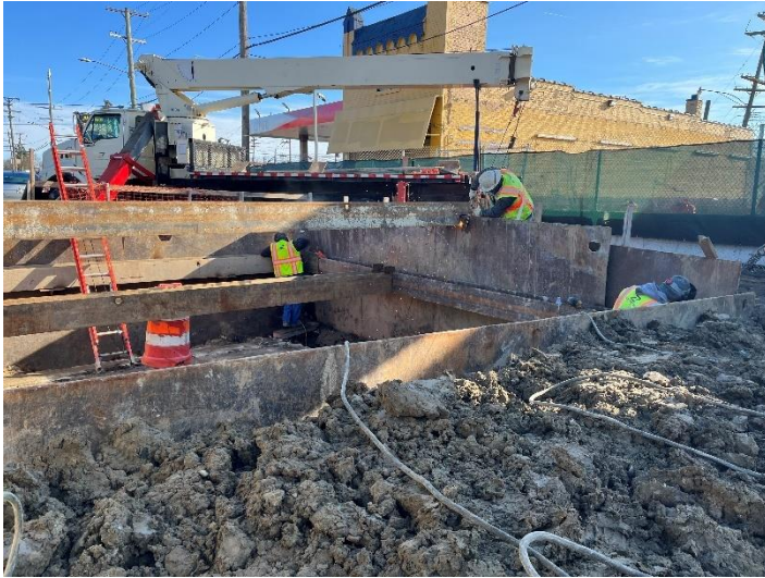
Contractor installing upper walers for TERS
