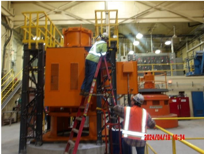
Contractor filling motor and bearing oil at Pump #5
