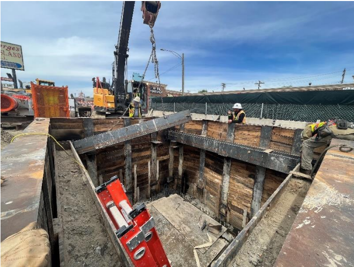
Removal of bracing from the east side of the access shaft
