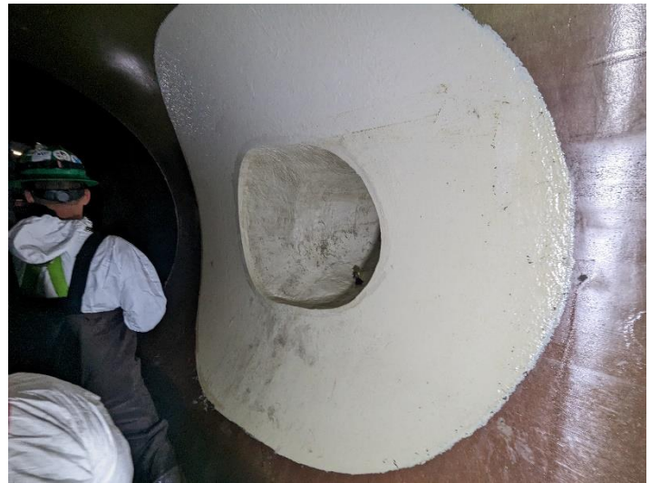
Epoxied ST-S-5 connection
