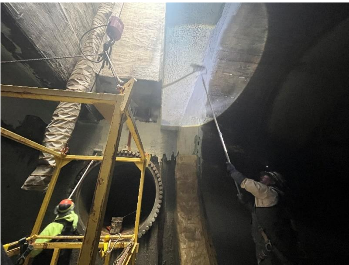
The application of Mainstay 714 coating in discharge chamber
