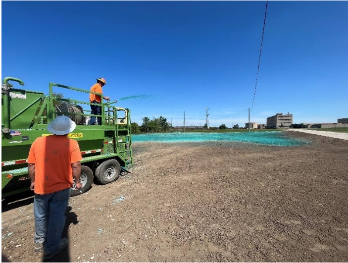
Restoration of laydown yard via hydroseeding
