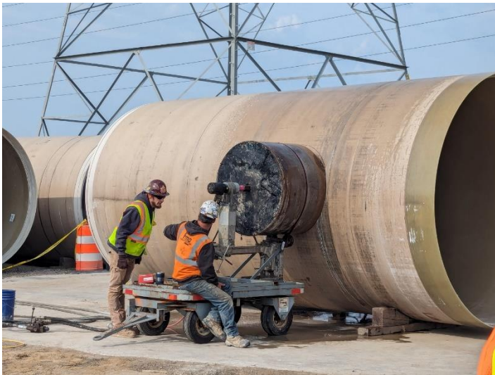
Preparing Hobas pipe section for lateral connection
