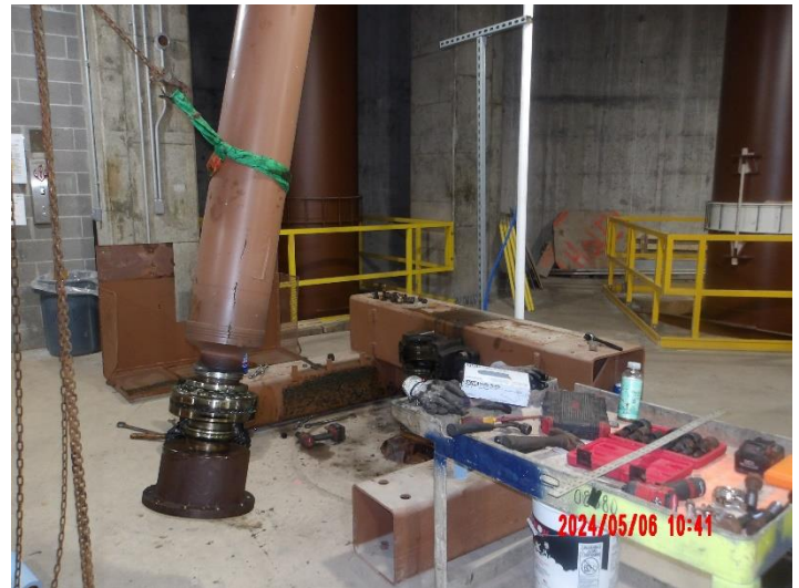
Installation of new Pump #4 shaft bearing for Pump #4
