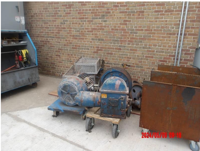
Part of the demolition process of the existing elevator
