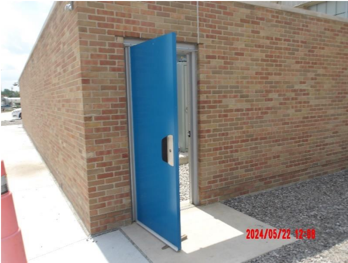
Newly painted doors to transformer enclosure
