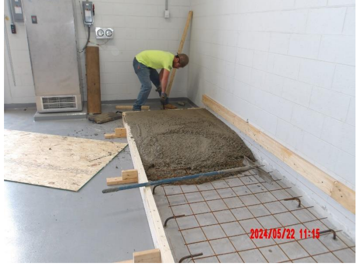
Pouring concrete pad for Pump #4 VFD panel
