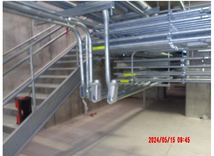
Installation of electrical conduits for Pump #4
