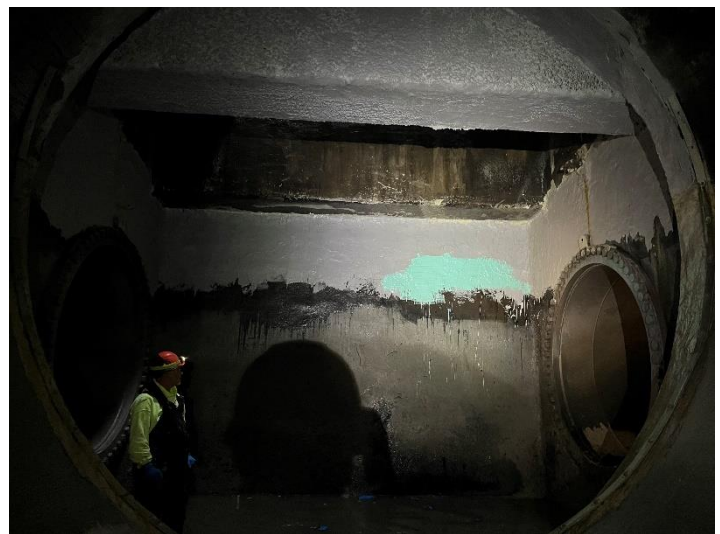
Application of Quadex Structure Guard for repair
