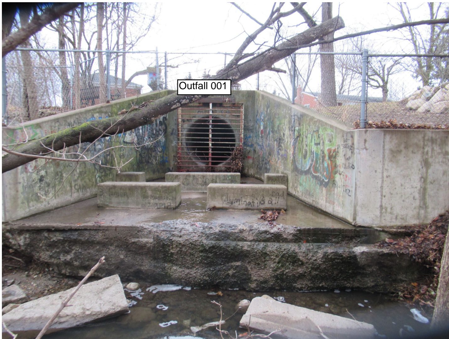
Enclosed portion outlet (001) downstream of Hutton Street.
