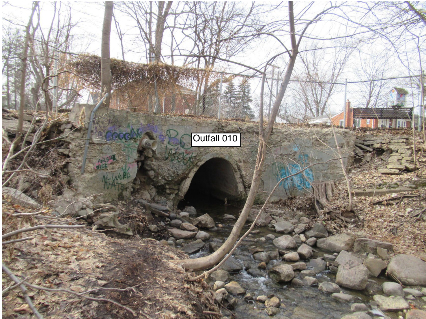
Hutton Street culvert over low flow channel.
