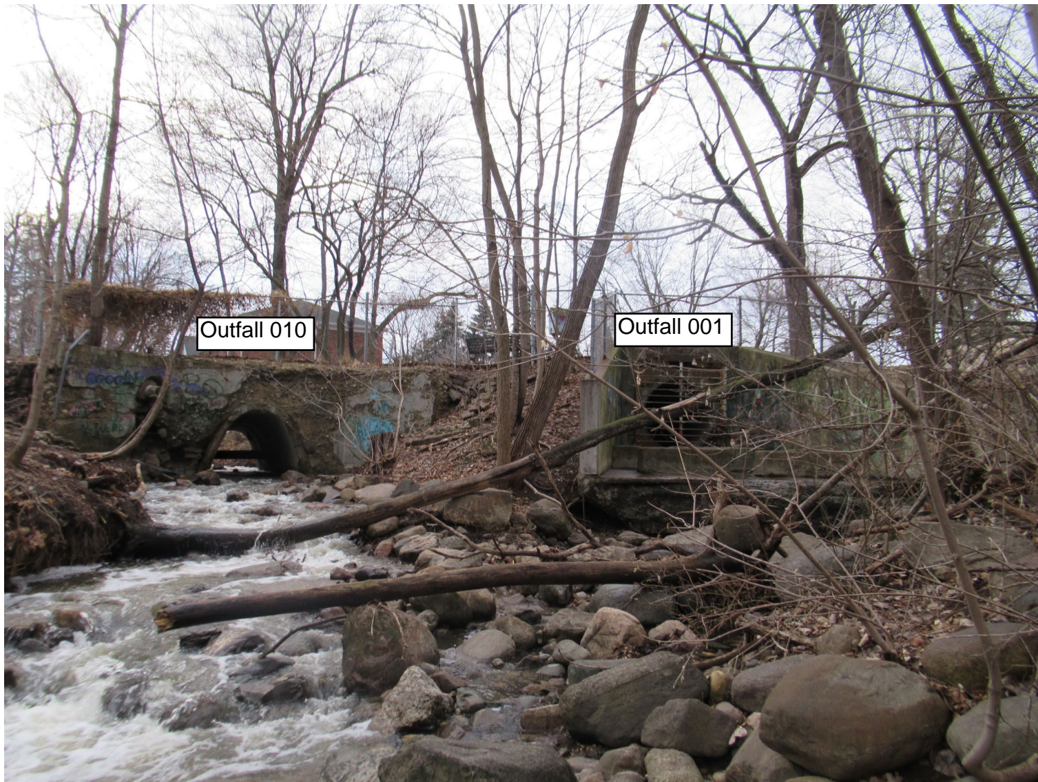
Downstream terminus, looking upstream toward Hutton Street.
