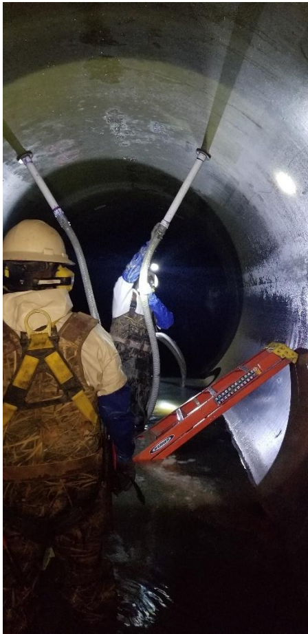
Annular grouting operations
