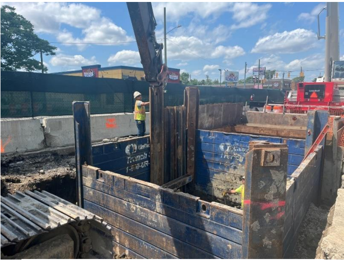
Slide-rail Earth Retention System
