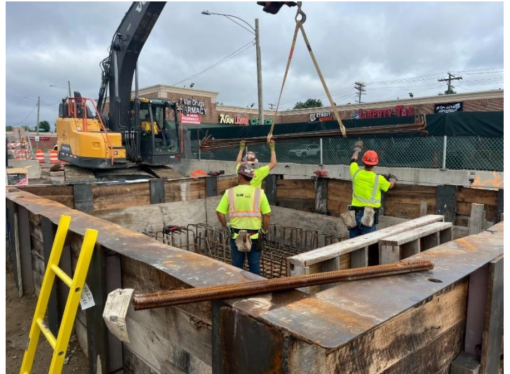
7 Mile access shaft top slab reinforcement
