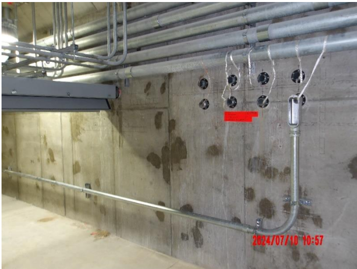
Contractor pulling 480 volt lines from electrical switchgear
