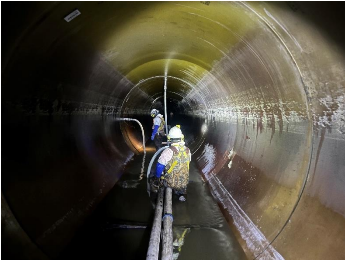
Grouting annular space of installed Hobas
