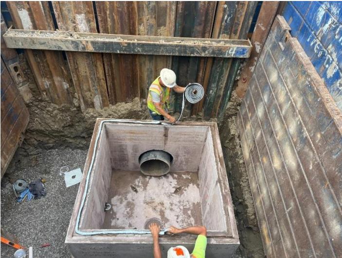
Receiving pit near PC663
