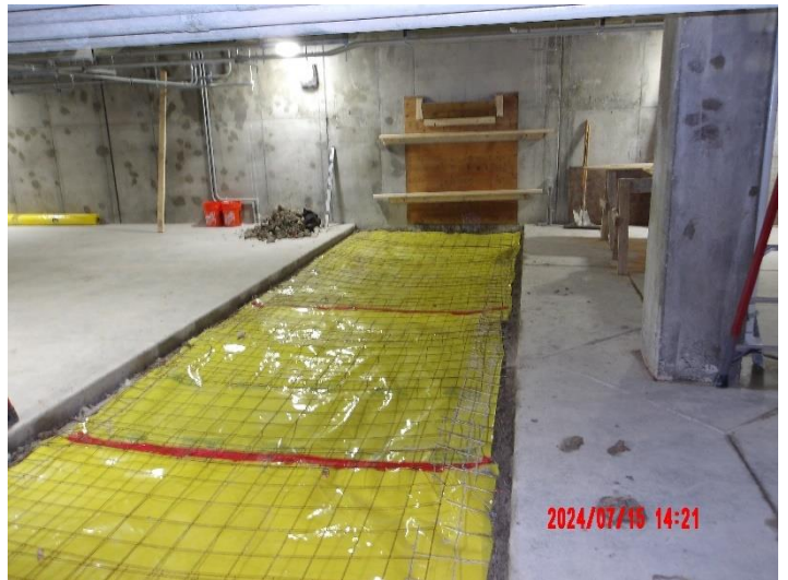
Pouring the basement floor strip
