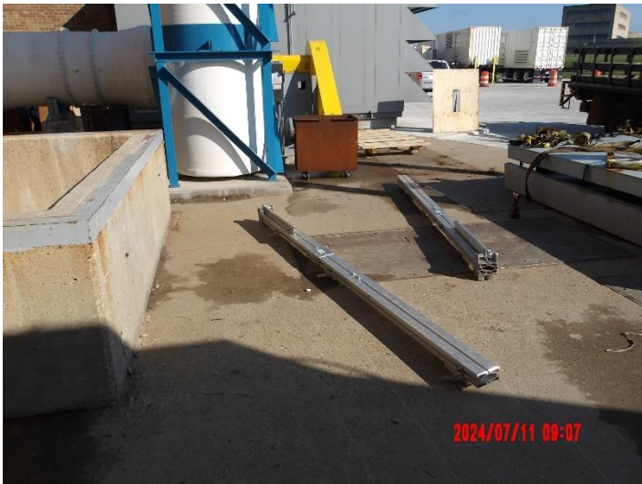
New tracks for wet well elevator
