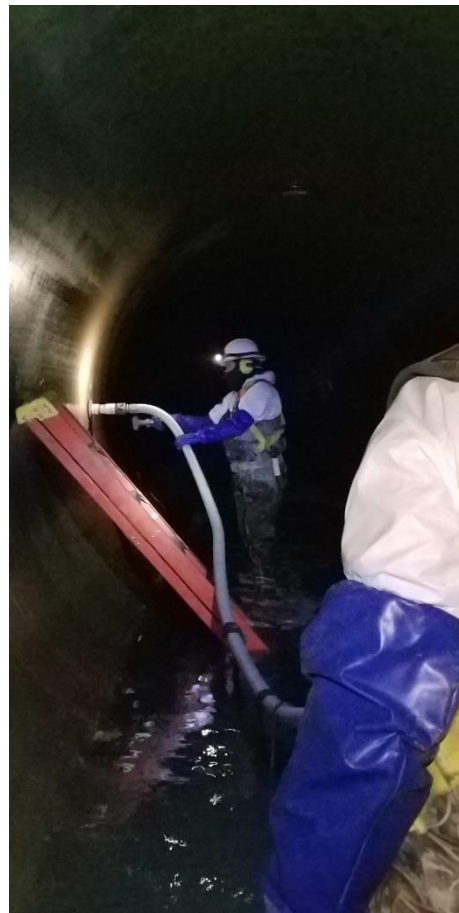
Annular grouting operations
