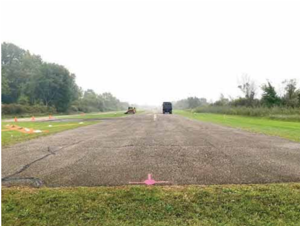
Photo 4. Conditions in Runway 8 APE, facing east
