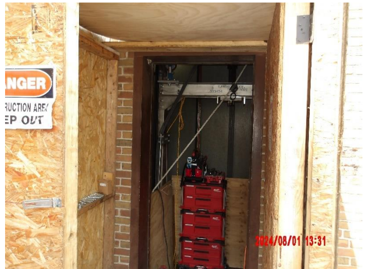
Wet well elevator under construction
