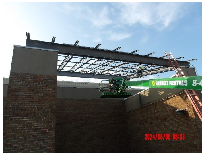
Installing outside shed roof
