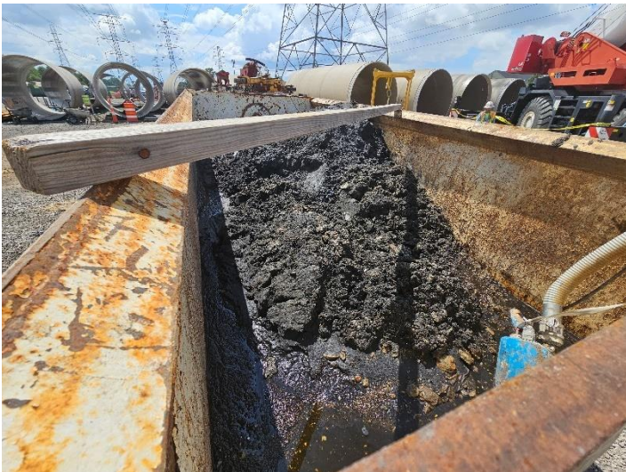
Debris removed from sewer decanting topside
