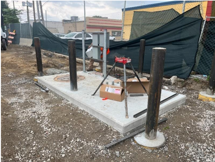
Installation of meter enclosure
