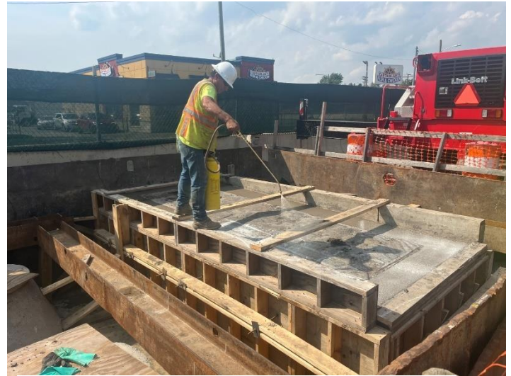
Pouring and curing of PC-663 vertical section
