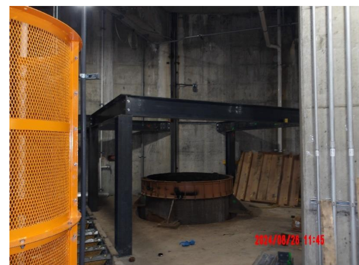
Removing Pump #6 magnetic flow meter platform
