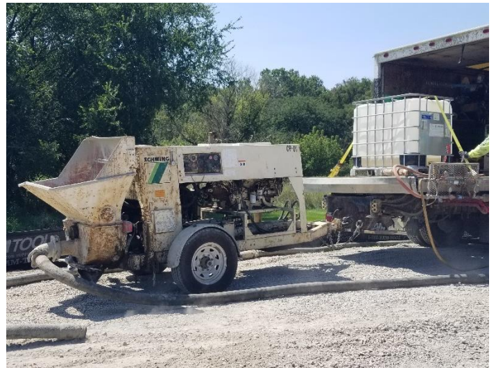
Manhole grouting set-up at MH-1
