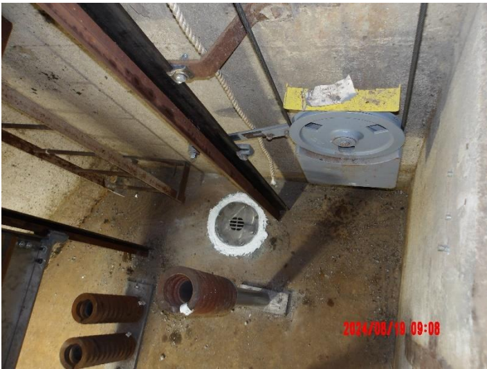
Construction of floor drain for wet well elevator pit
