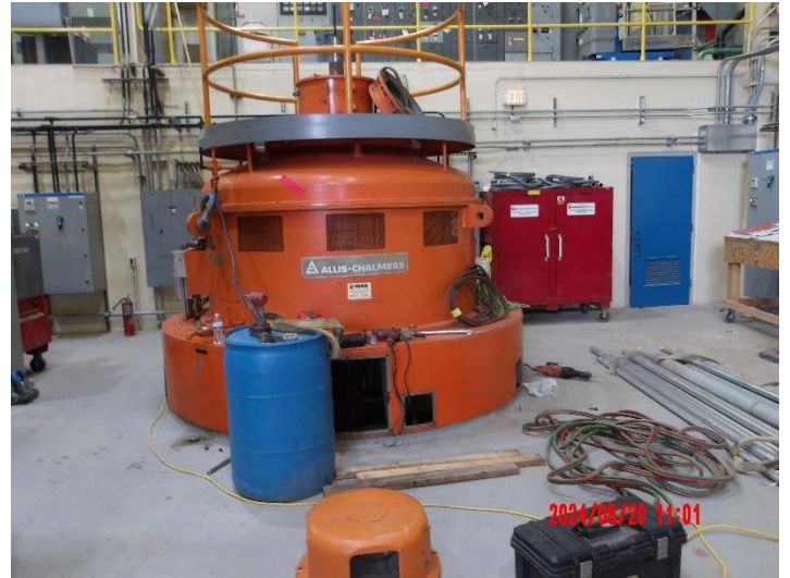
Preparing to demolish Pump #6 electrical motor
