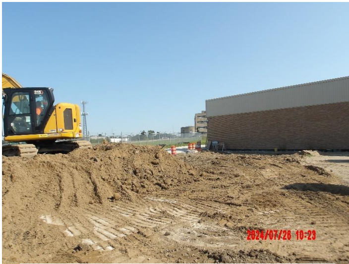
Hauling away spoils from duct bank trench
