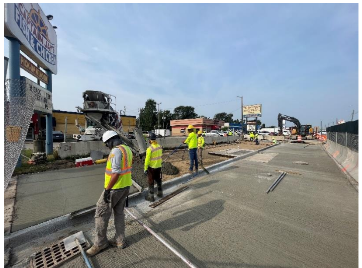
Restoration of road and sidewalk
