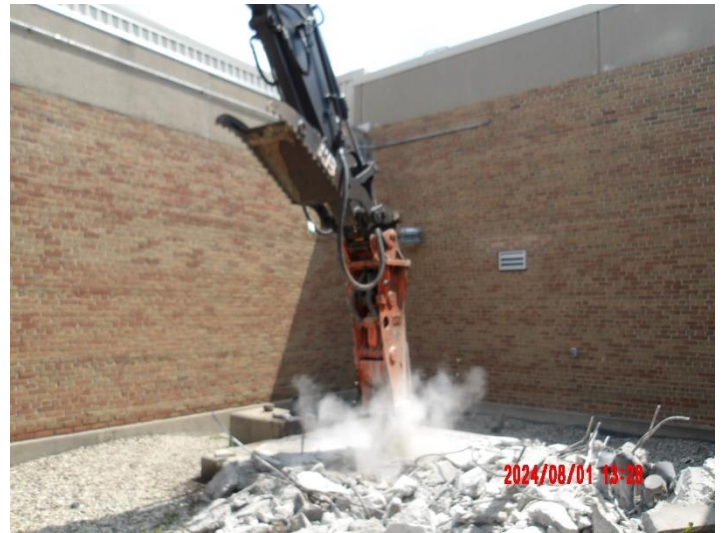
Demolition of existing Transformer foundation
