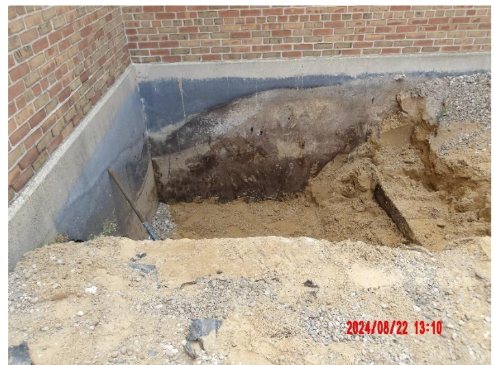
Restoring grade north of existing Transformer enclosure
