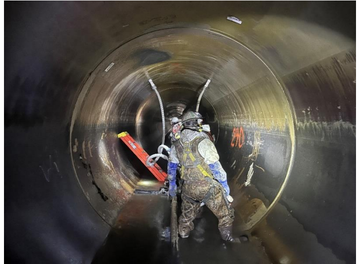
Grouting efforts at Hobas section 240
