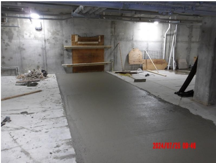
New concrete floor in electrical building basement
