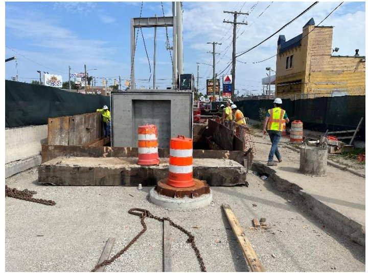
Installing bulkhead gate
