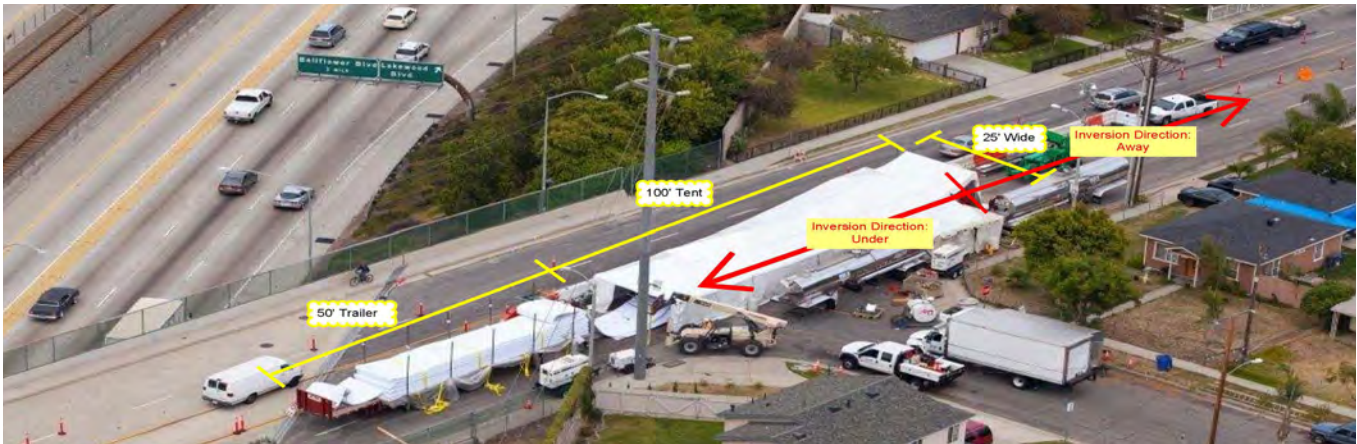
Figure 10. Over-The-Hole OTH set up with lengths and inversion direction
