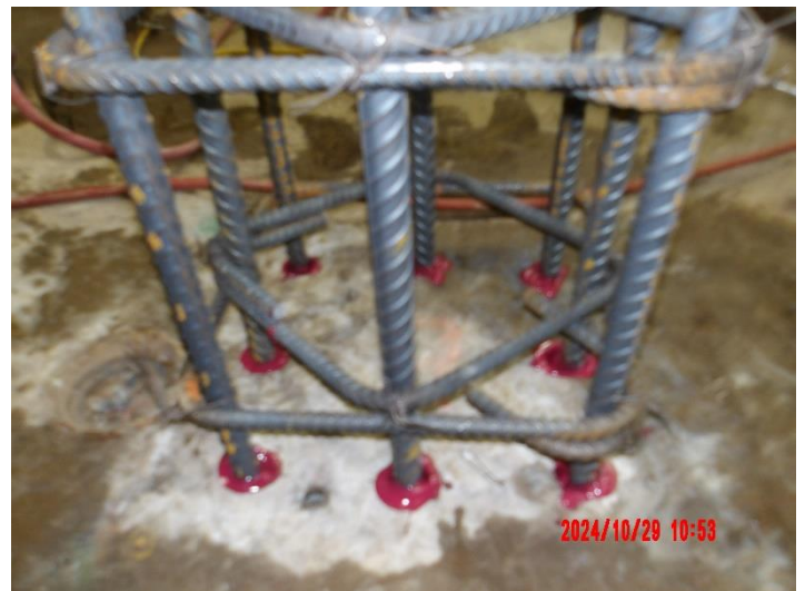
Pump #6 support install (upper and lower)
