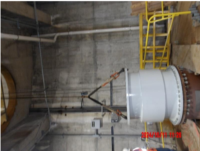
Installing Pump #6 magnetic flow meter
