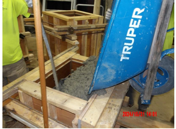
Pump #6 support install (upper and lower)
