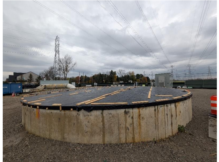
Temporary roof for CS-12
