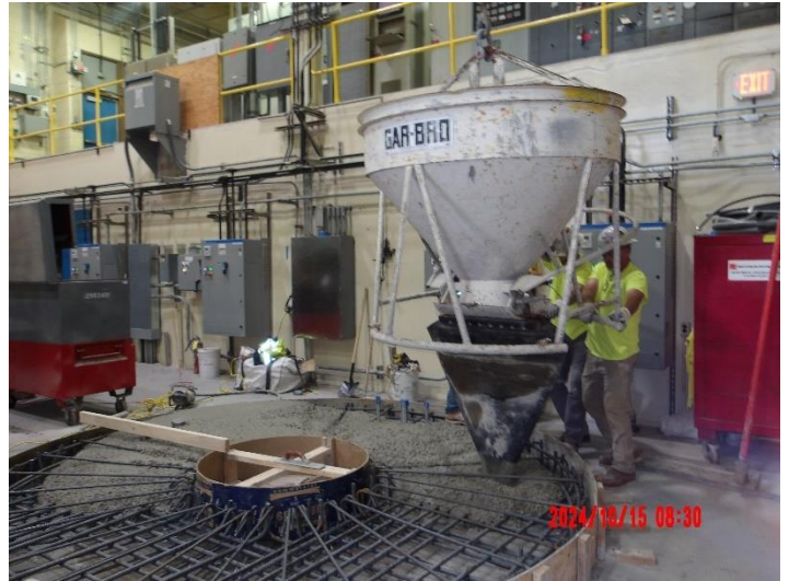
Preparing pump #6 discharge pipe for installation
