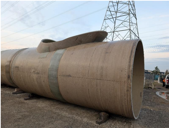
Stage slip-lining pipe segment
