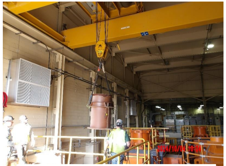
Pouring Pump #6 electrical motor footing
