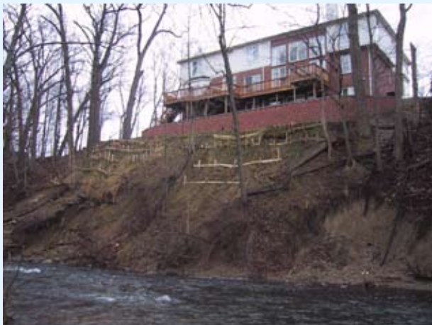
This house is threatened by erosion of the banks along the Clinton River as the river works to stabilize itself in response to increased loads of water and sediment from its watershed.
