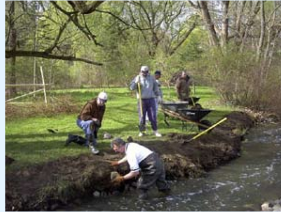
Pebble Creek Stabilization Project
