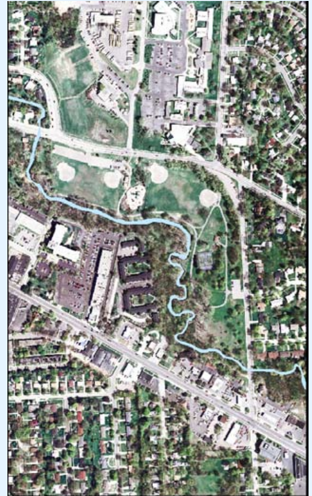
This area of the Rouge River is impacted by intense surrounding land uses and narrow buffer vegetation.
