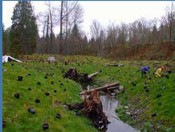
EPA Five Star Streambank Stabilization effort
