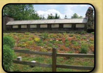
Green Roofs Addison Township
