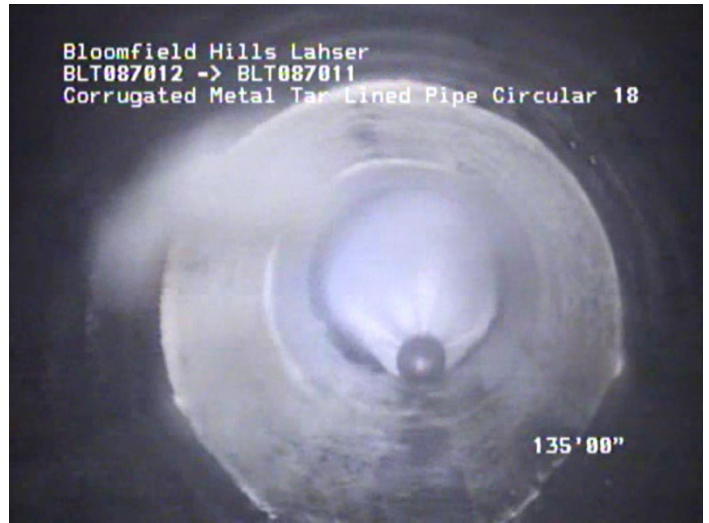
Existing Pipe Patch Rehab
