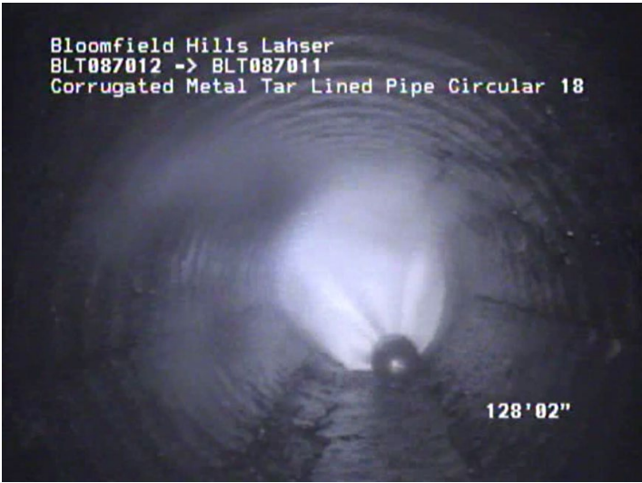
Deteriorated Invert
