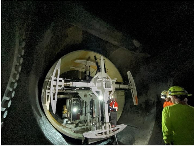
Installing Initial (Transition) Pipe Section
