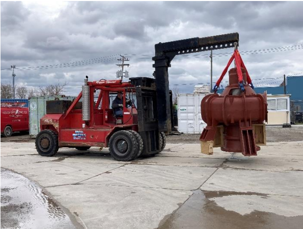
Delivery of Sanitary Pump #1 on April 19, 2022
