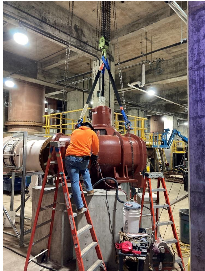
Positioning Sanitary Pump #1 on April 28, 2022
