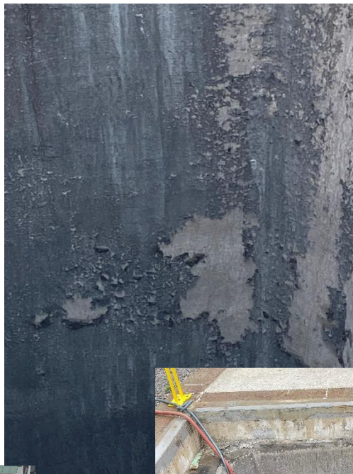
Peeling Surface Coating of NESPS Central Discharge Chamber (Below and to Left)
