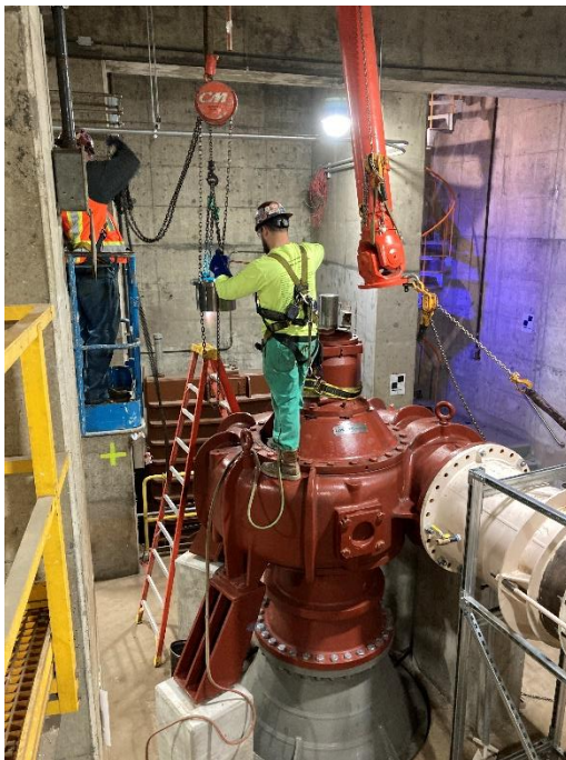
Pump 1 Shaft Coupling Installation
