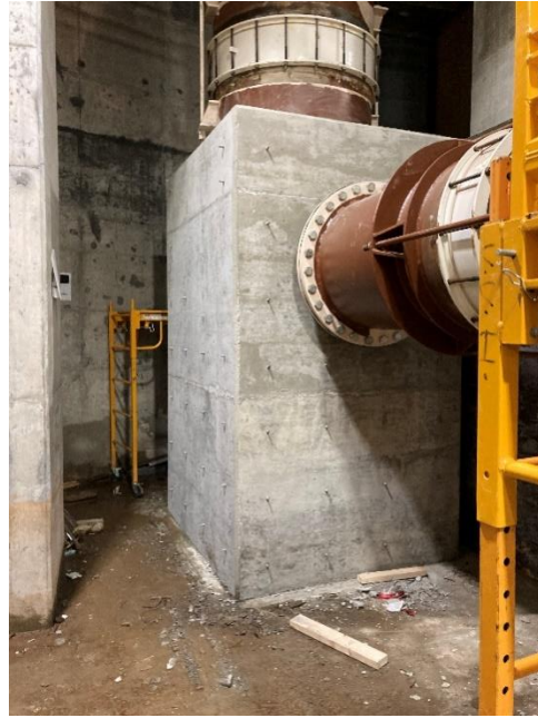
Completed Pump 3 Thrust Block
