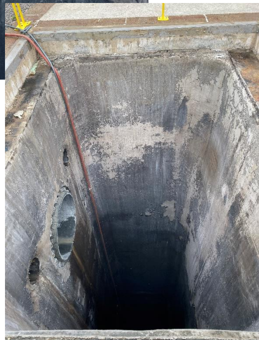
Peeling Surface Coating of NESPS Central Discharge Chamber (Below and to Left)
