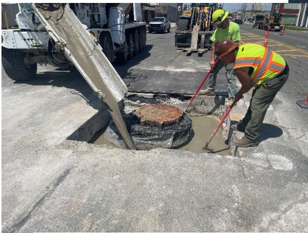
Manhole Cone Replacement on Van Dyke
