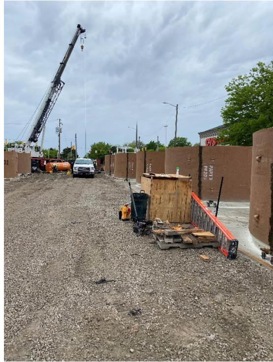
Channel Line Sections Assembled and Ready for Installation
