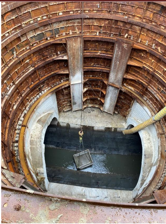
Access Shaft Clean and Ready for Pipe Installation
