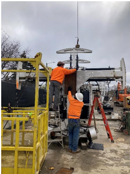
Installation of Reinforcement on Pipe Carrier
