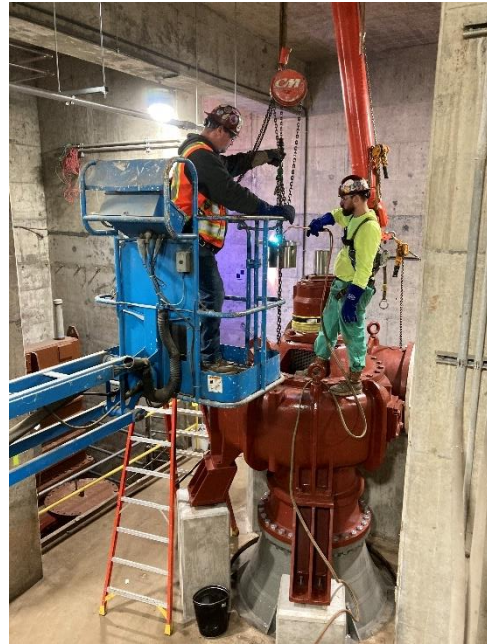
Pump 1 Shaft Coupling Installation
