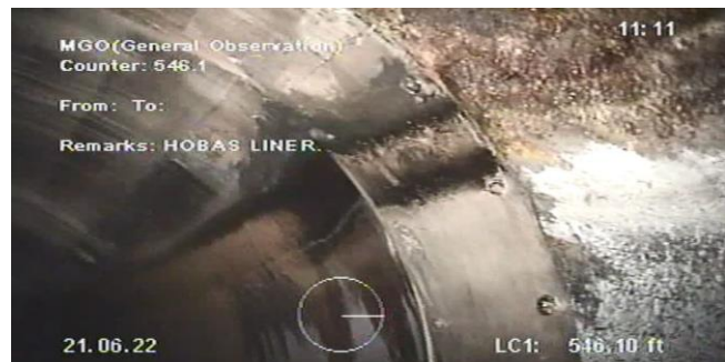
Hobas liner between PCI-7-17A and PCI-7-108
