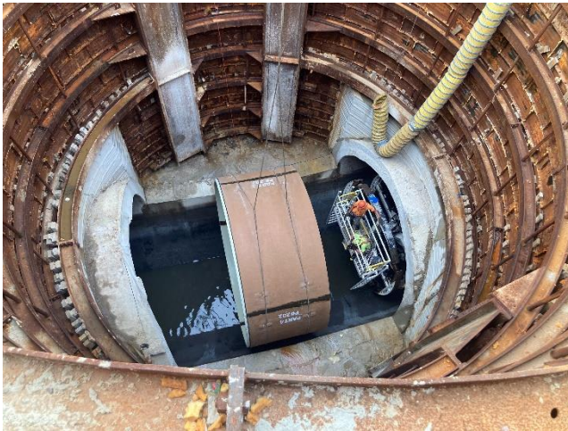
Channeline pipe being lowered into the Interceptor
