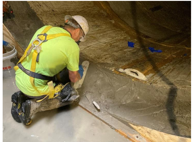
Work on Discharge Chamber taper transition
