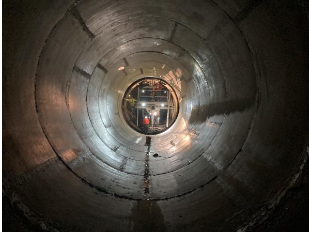
View downstream of Channeline pipe installed
