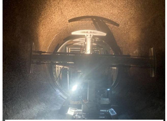
Channeline pipe placement from behind pipe carrier
