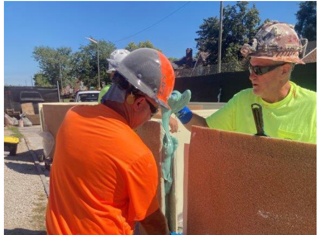
Application of Crestabond to Channeline for assembly
