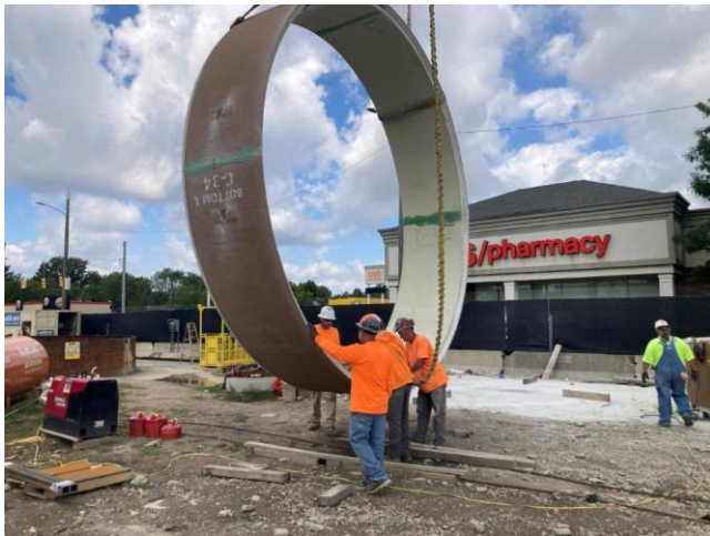
Marra positioning Channeline for placement in Interceptor
