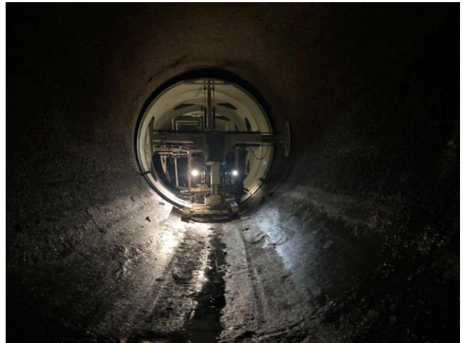
Marra installing Channeline pipe sections through curve of interceptor
