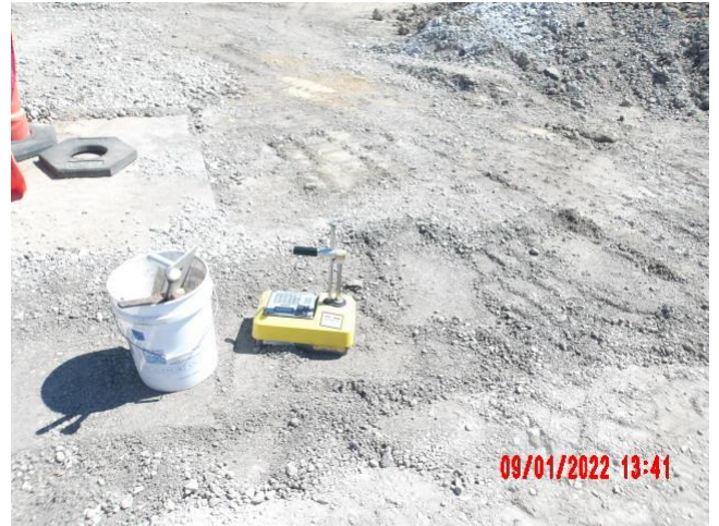
Density testing of backfill for new fiber optic duct-bank
