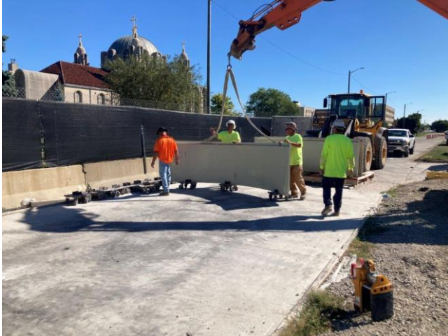
Channeline pipe placement from behind pipe carrier
