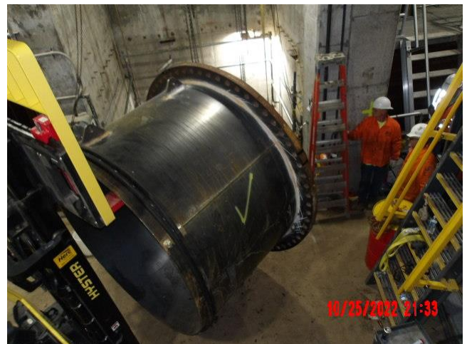
Installing temporary spool piece
