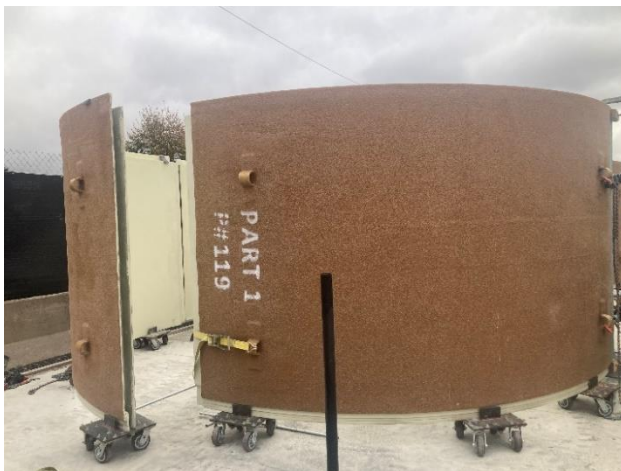
Continued assembly of Channeline pipe on October 17, 2022
