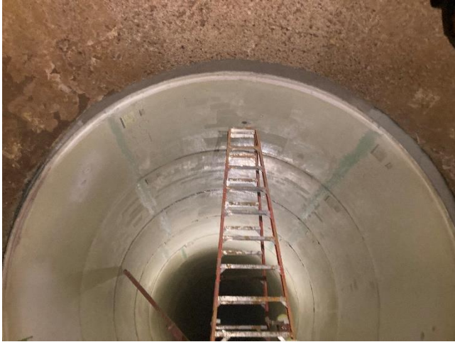
Grouting bulkhead of Channeline pipe section P#123
