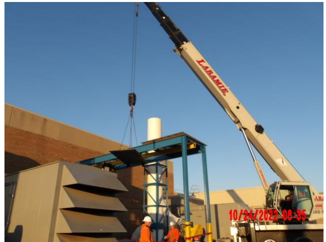
Placing stop log before removing KGV #2
