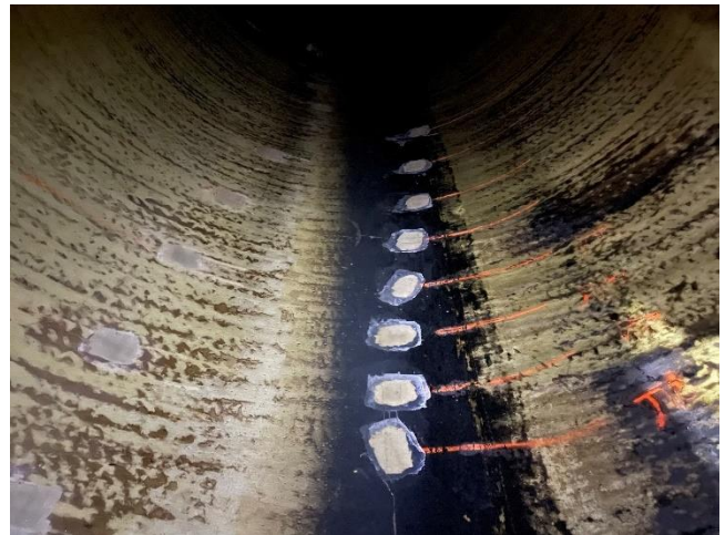
Repairs of Hobas underway at CS-9 in early October 2022
