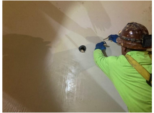
Installation of grout ports and vents for annulus grouting
