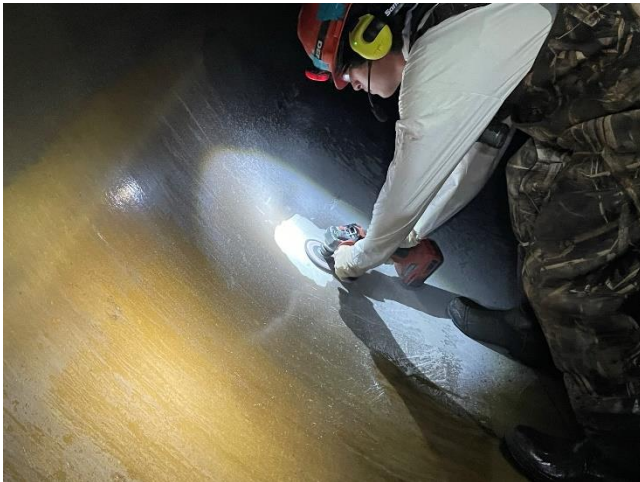
Repairs of Hobas underway at CS-9 in early October 2022
