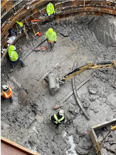
Removing wood lagging from PCI-4 in early December 2021
