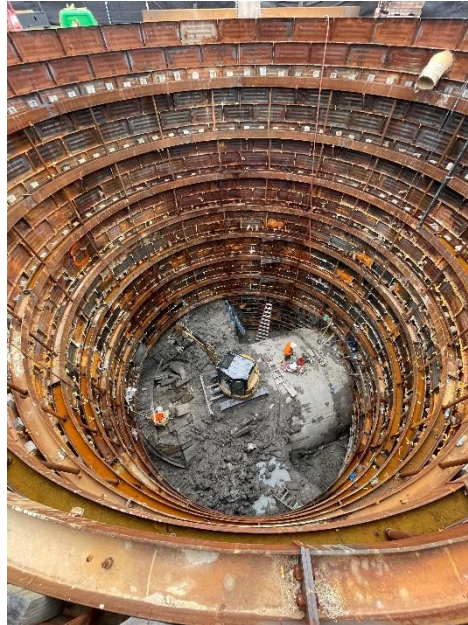
Status of excavation in mid-December, 2021
