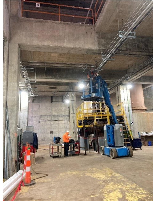
Ongoing splicing within manhole MH E9A
