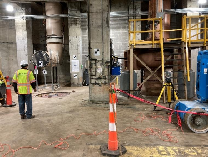
3D capture to verify pump orientation
