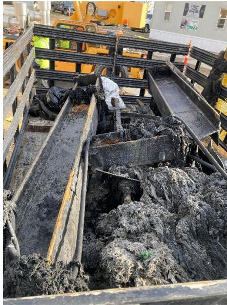
Debris cleaned from downstream of PCI-4, including structural steel from original gatehouse discharge piping support frames
