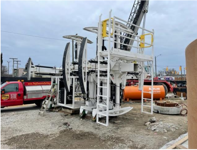
Pipe carrier on-site
