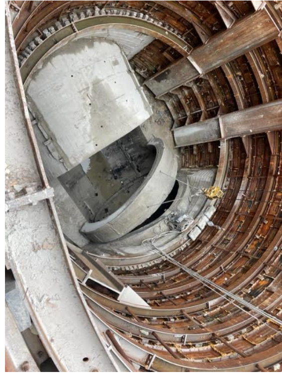
Removing crown of the Interceptor
