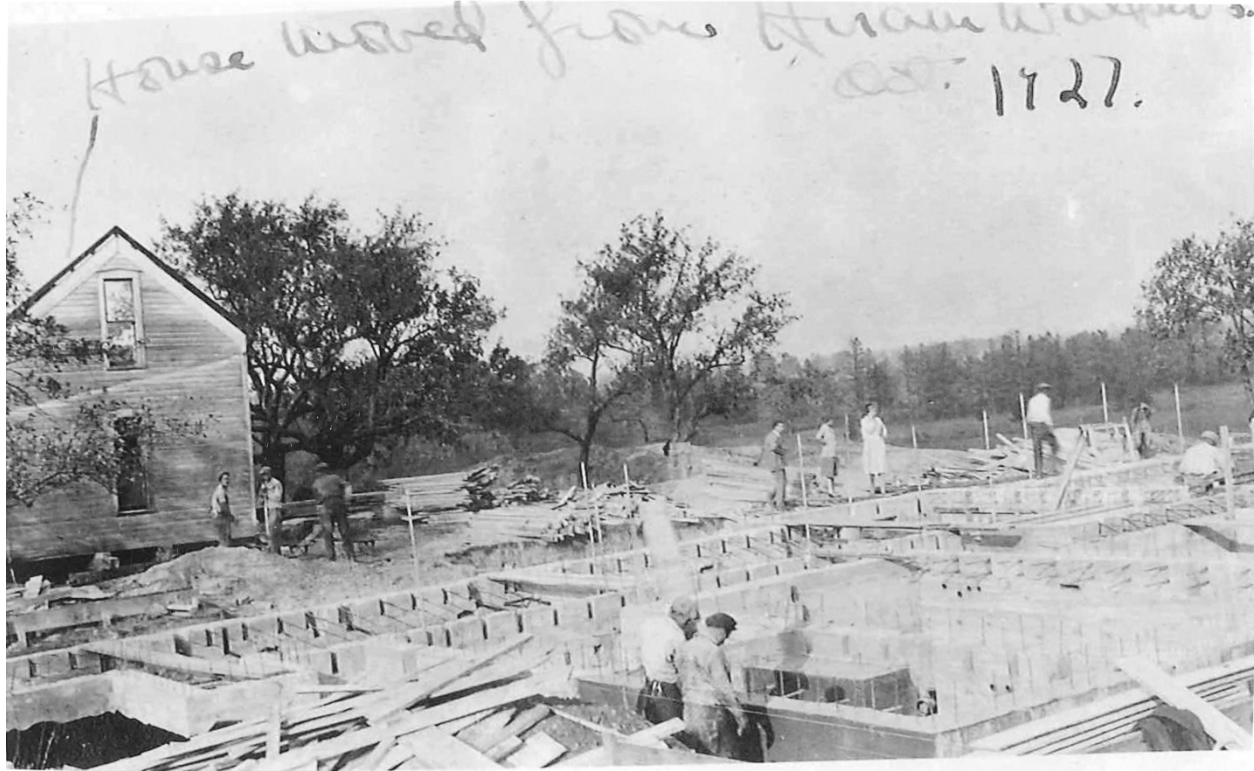
Photo: Construction of the Buhl home (current Conference Center) in 1927
