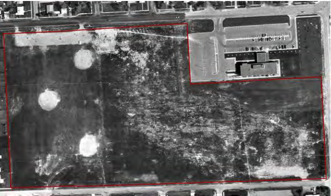
◀ 1974 Aerial Photo with current park boundary overlay indicating the Southfield Little League ball fields and parking lot in proximity to the Oakland County Health Department
