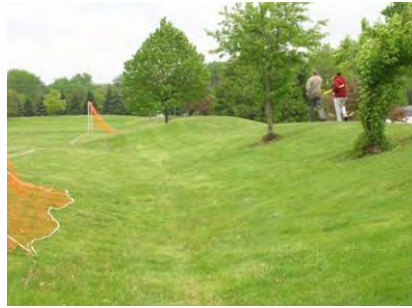
▲ Swale and Turf Drain
