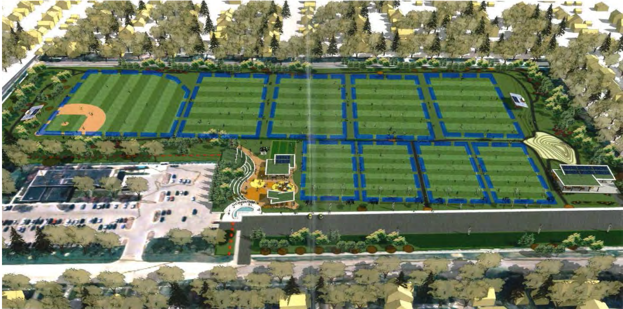
Catalpa Oaks Overview (Barton Malow, 2010), looking south
